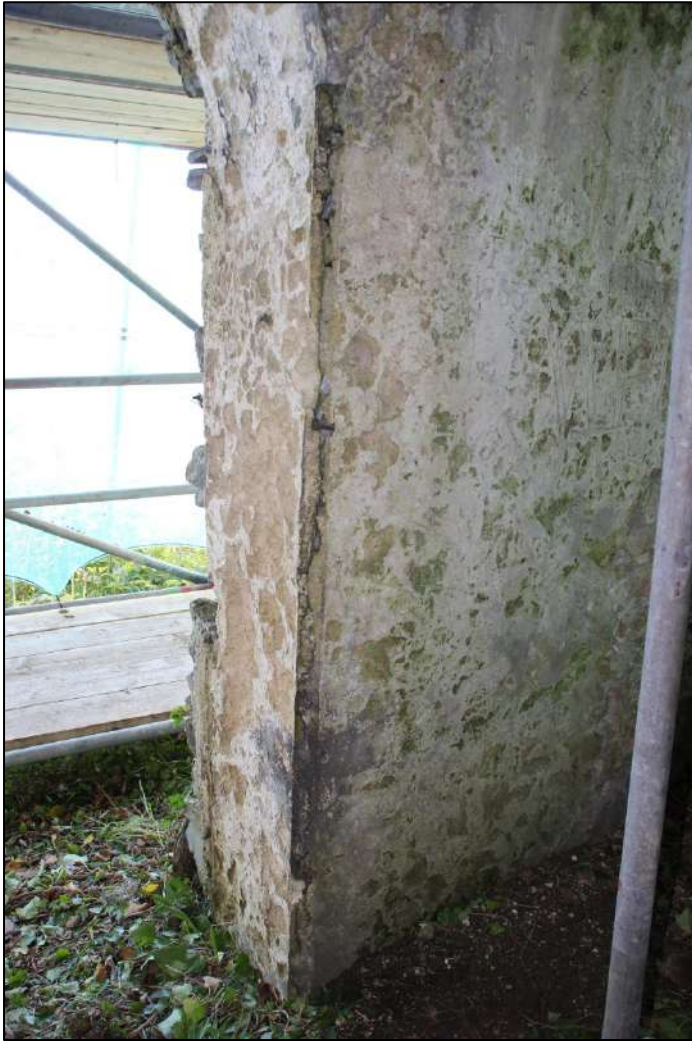
Pl. 23 This is the southern side of the main entrance where the impression of the corner beading can be seen.
