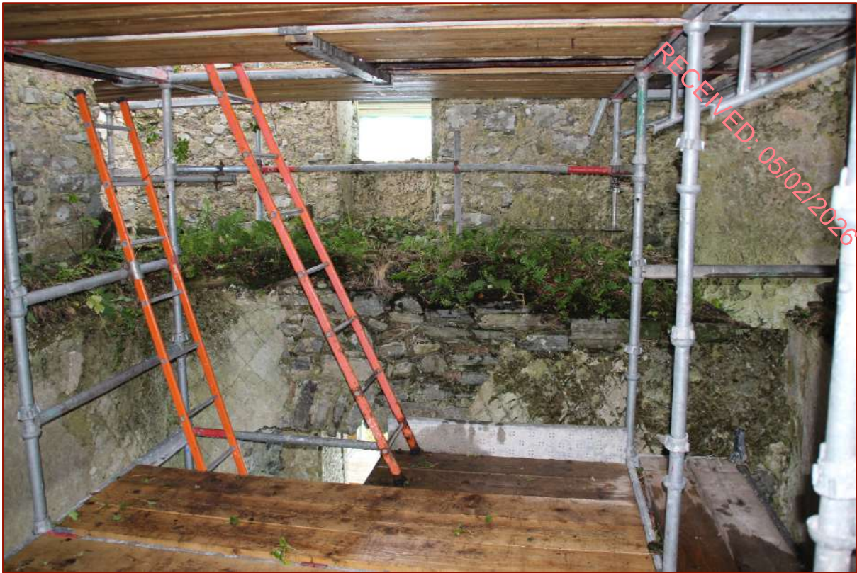
Pl. 6 The eastern end of the ground floor chamber. There may have been a partition wall where the vegetation is growing. No coving survives below that level. The stairs is on right.
