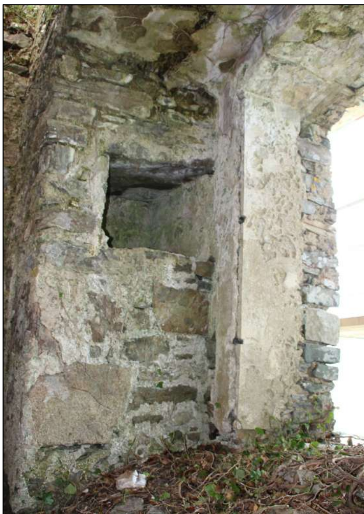
Pl. 22 Southern side of western window embrasure, first floor. Note the impression of a timber corner bead on the inner side of the reveal. The holes on the edge mark where timber plugs were used to attach the beading to the stonework.
