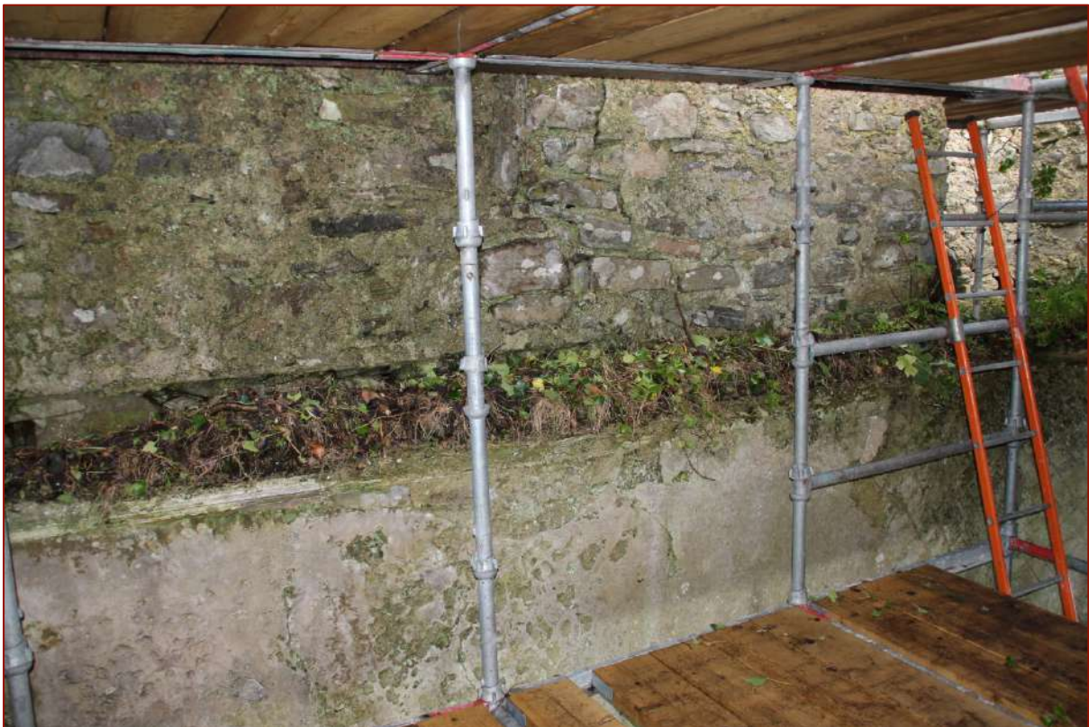
Pl. 5 The coving on the north wall of the main chamber of the ground floor. The band of vegetation across the centre marks the position of the ceiling of the ground floor and floor of the first floor. Only the portion on the western side (on left) survives to any extent.
