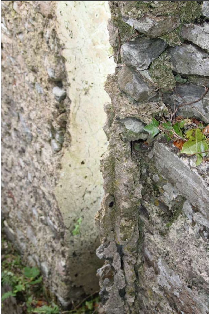
Pl. 21 Impression of a timber upright in the plaster on the southern side of the eastern window at first floor level. The wall on the left of the window is thinner, having been rebuilt.
