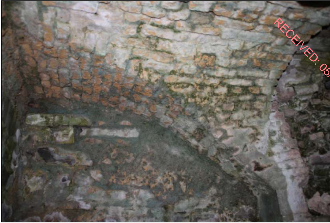
Pl. 139 The brick groin vaulting in kiln 2.
