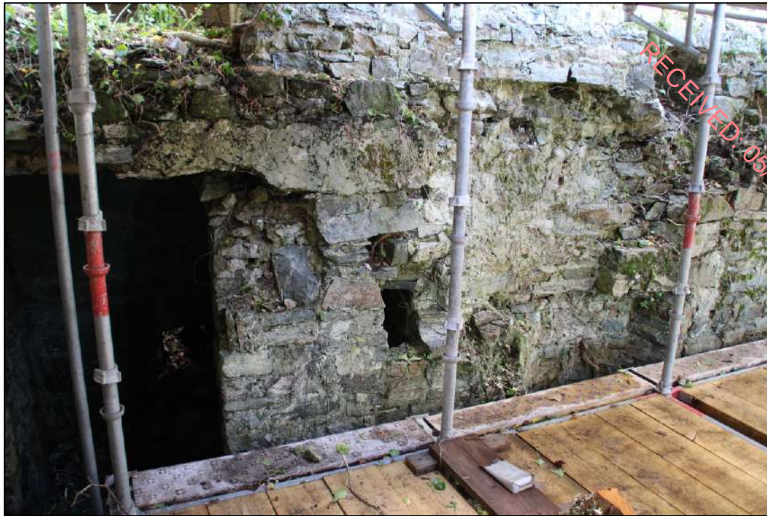
Pl. 126 The south-western side of the large room of the industrial building. The doorway leads to kiln 1. Immediately right of the ope at the centre of the photograph is a shallow fireplace.
