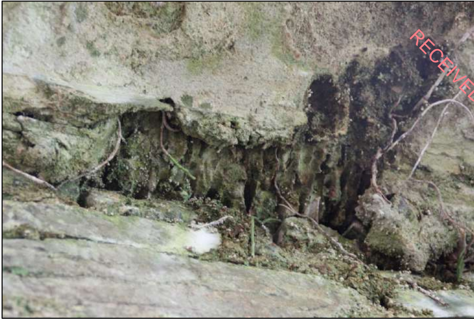
Pl. 86 Impression of wickerwork centring, southern side of the western window embrasure, first floor.
