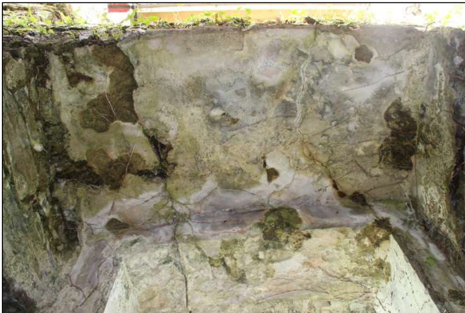
Pl. 85 View of the plastered soffit of the western window embrasure. Traces of the impression of wickerwork centring are present on the extreme left.
