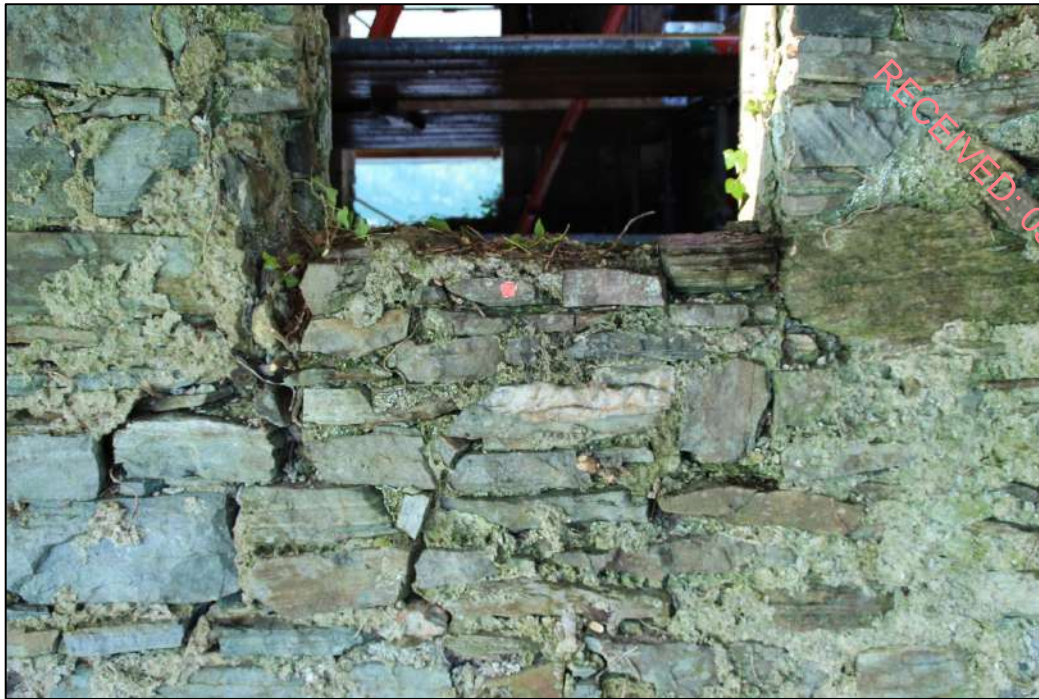
Pl. 9 Infilled area at base of window
