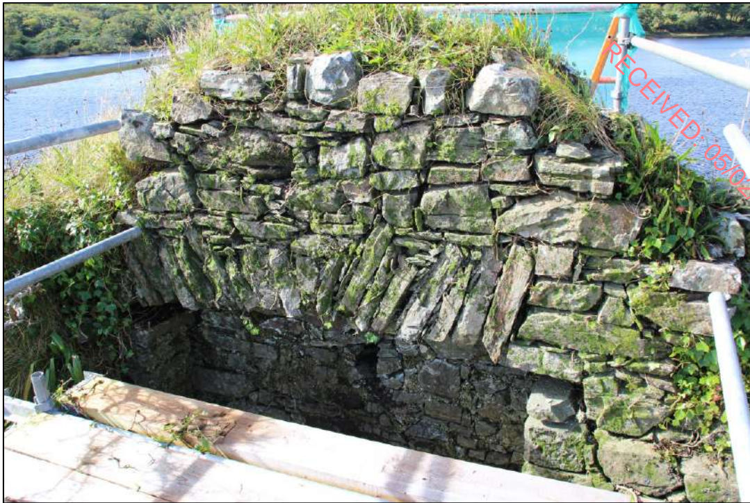
Pl. 96 The upper part of the western gable showing the flat-headed arch over the window embrasure. A timber lintel supported the arch.
