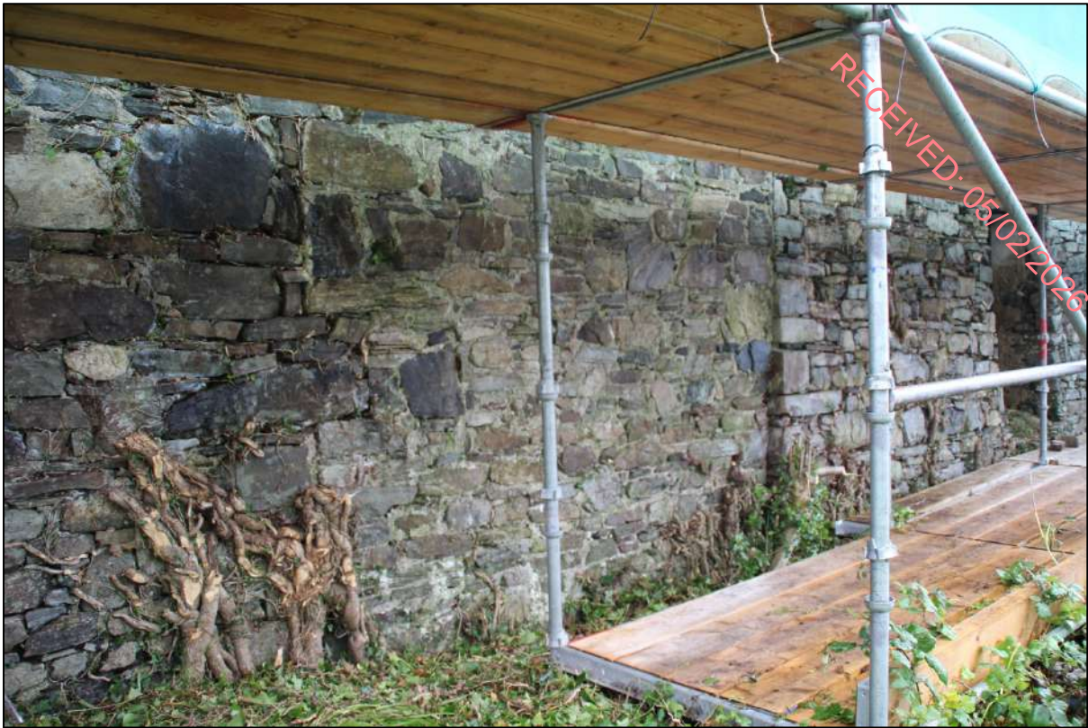
Pl. 31 The clear difference in the masonry of the central part of the wall marks the location of the first kiln erected on the site, kiln 1. The tower house is on the right and kiln 2 on the left.
