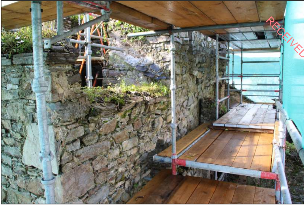
Pl. 13 The northern face of the tower house. The masonry on the left is all from the later rebuilding. Note the cornice at the top of the walls on left and the possible roof line or weatherslating at centre.
