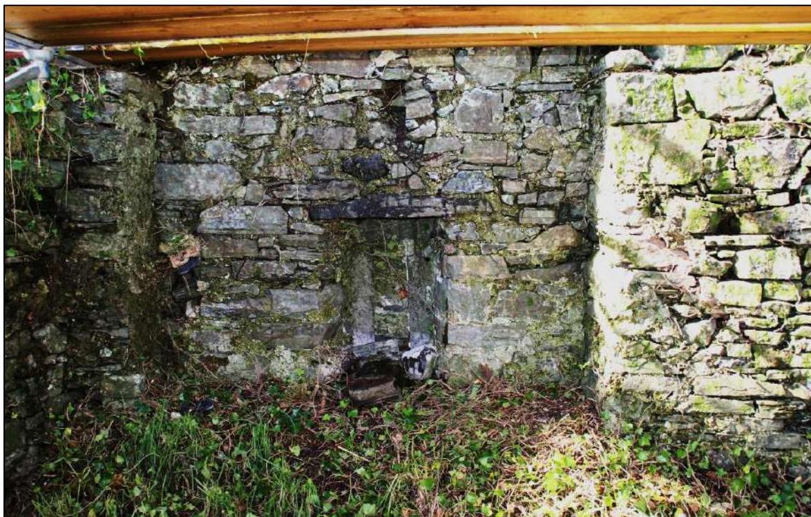
Pl. 97 The window embrasure on the western wall of the second floor. The window ope is blocked. There is a slot for a timber just above the window. Slight traces of a plaster scar are present on the northern (right hand) side of the embrasure. This extends from the slot downwards towards the inside of the northern and southern walls. It is very intermittent.
