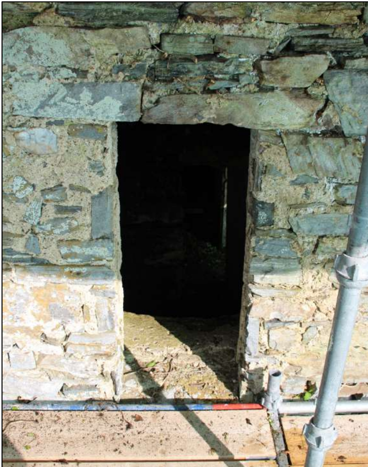
Pl. 36 This window lights the stairs and the entrance lobby. Southern elevation.
