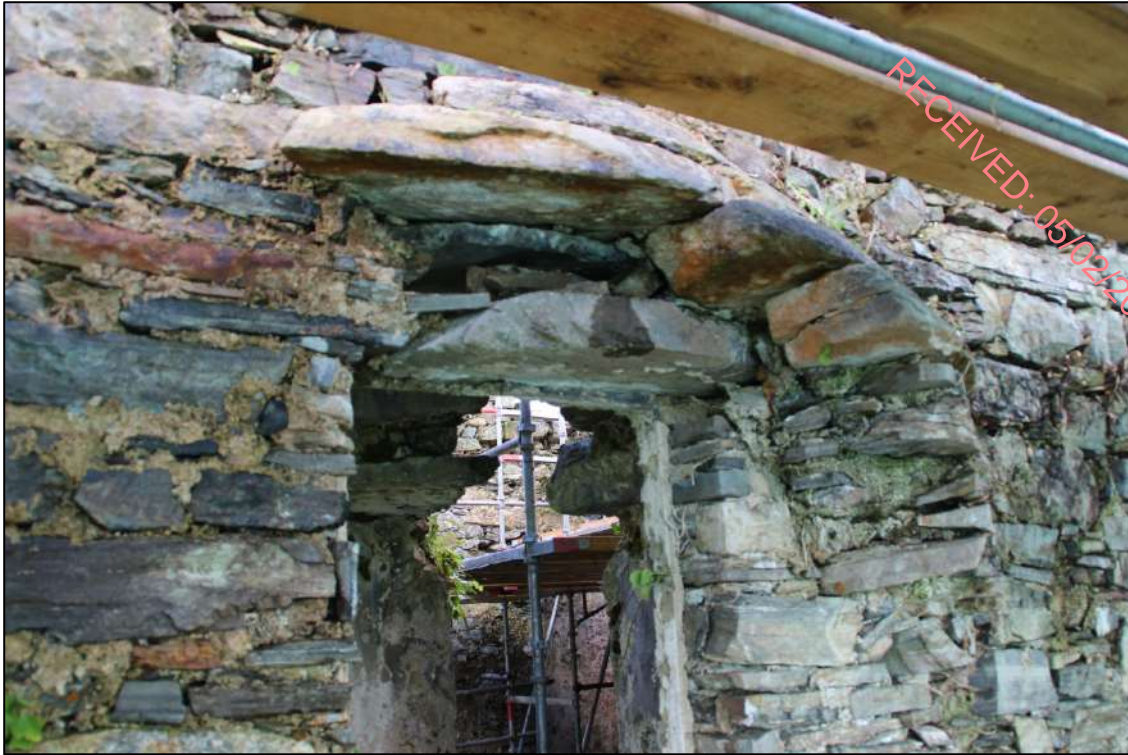
Pl. 25 Another view of the same hood. The unusual narrowing 'tail' still survives here.
