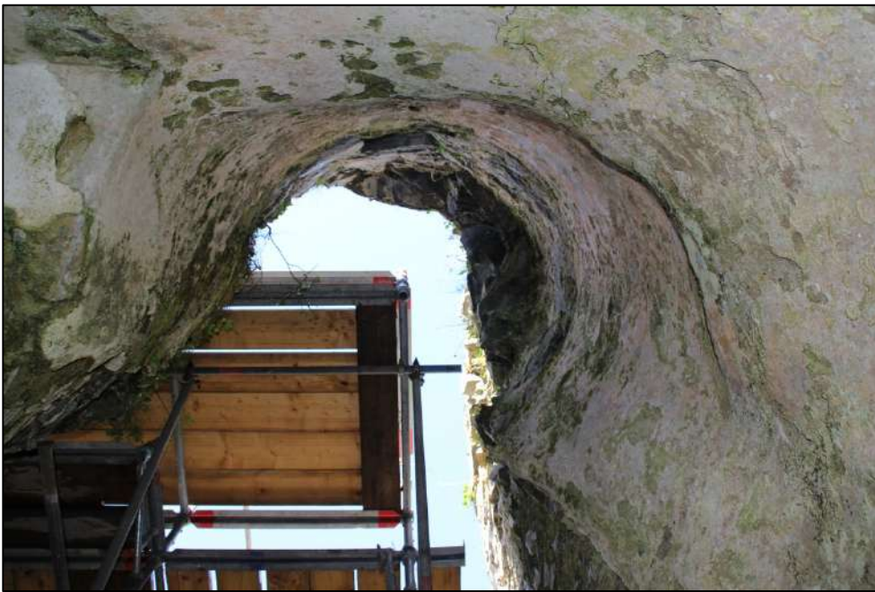
Pl. 63 Looking upwards at the stairwell from the highest remaining steps. It is likely that more were originally present, either in stone or wood. Note the good condition of the plaster finish.
