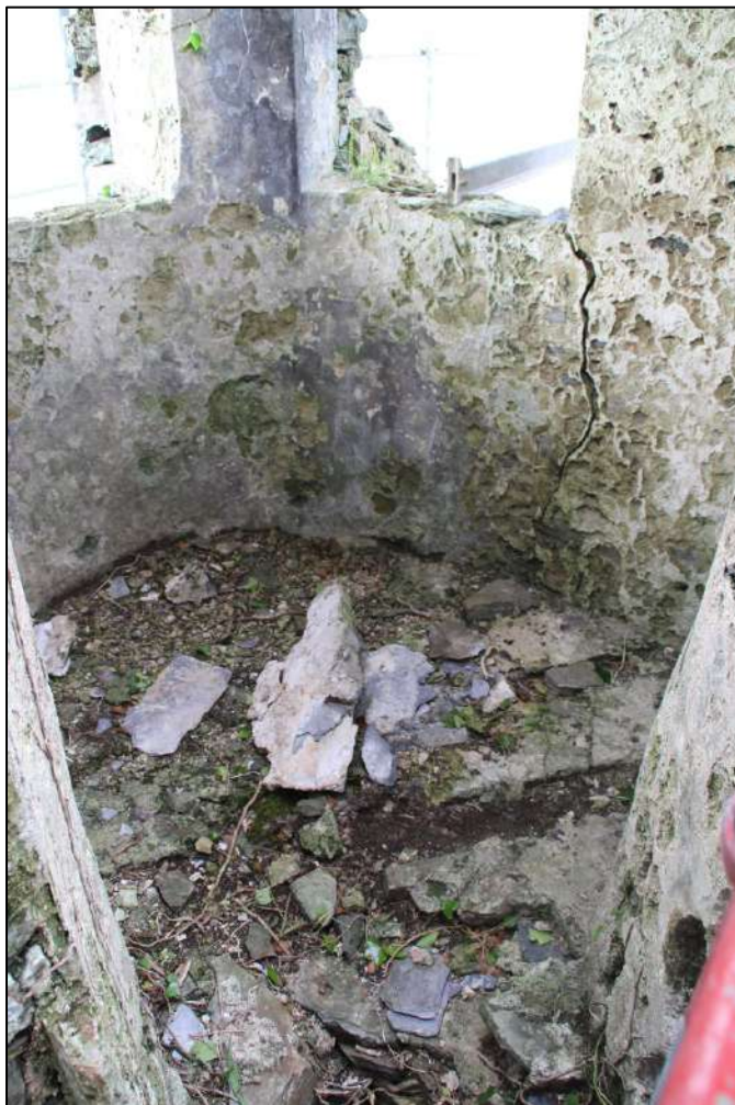
Pl. 93 The floor of the chamber. Note the linear slots which originally held timber boards. There are five in total. A timber floor would have been laid over these.
