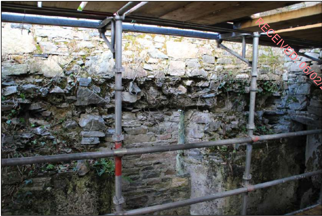
Pl. 122 Scar of the floor/ceiling line of the large room of the industrial building.
