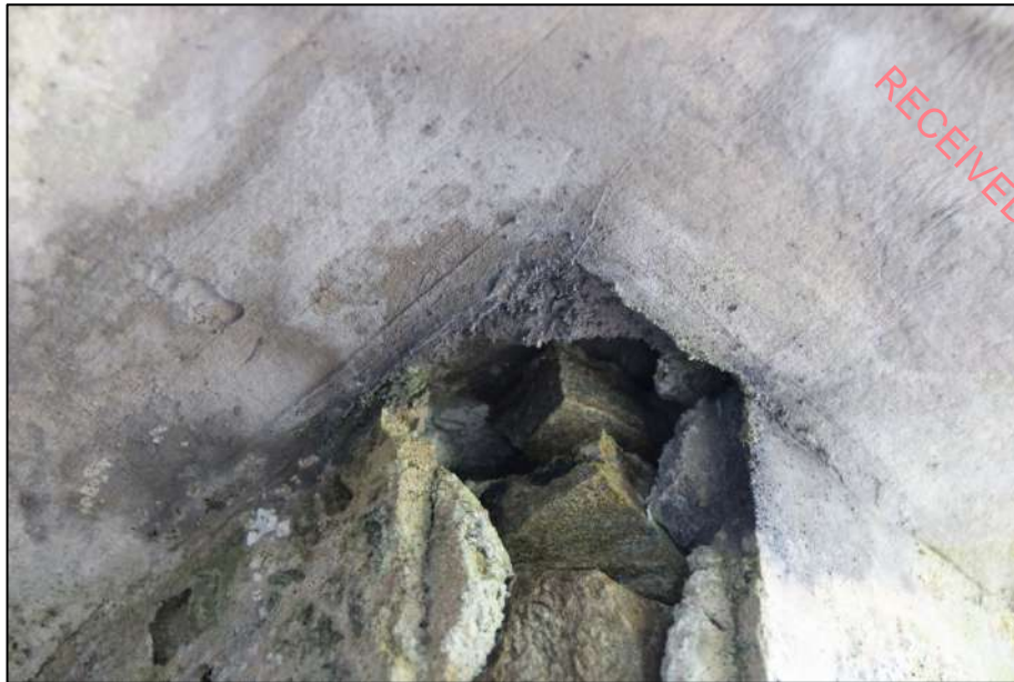
Pl. 52 Scar of the corner beading on the outer edge of the western embrasure on the ground floor
