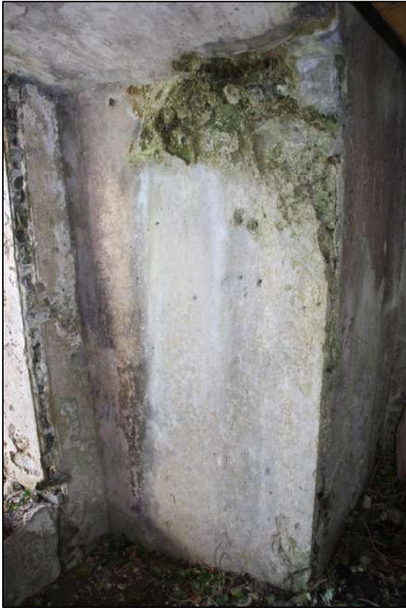
Pl. 54 Detail of the northern side of the embrasure. The centring impression is at the upper right.
