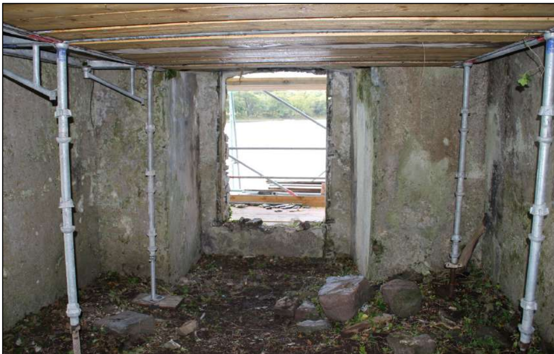
Pl. 53 The western window embrasure. Impressions of the wickerwork centring for the head of the embrasure survives in each upper corner.
