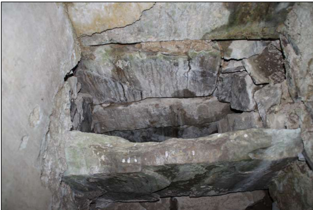
Pl. 69 Detail of the garderobe. Note that impressions of a timber seat or lid are on the left and right.
