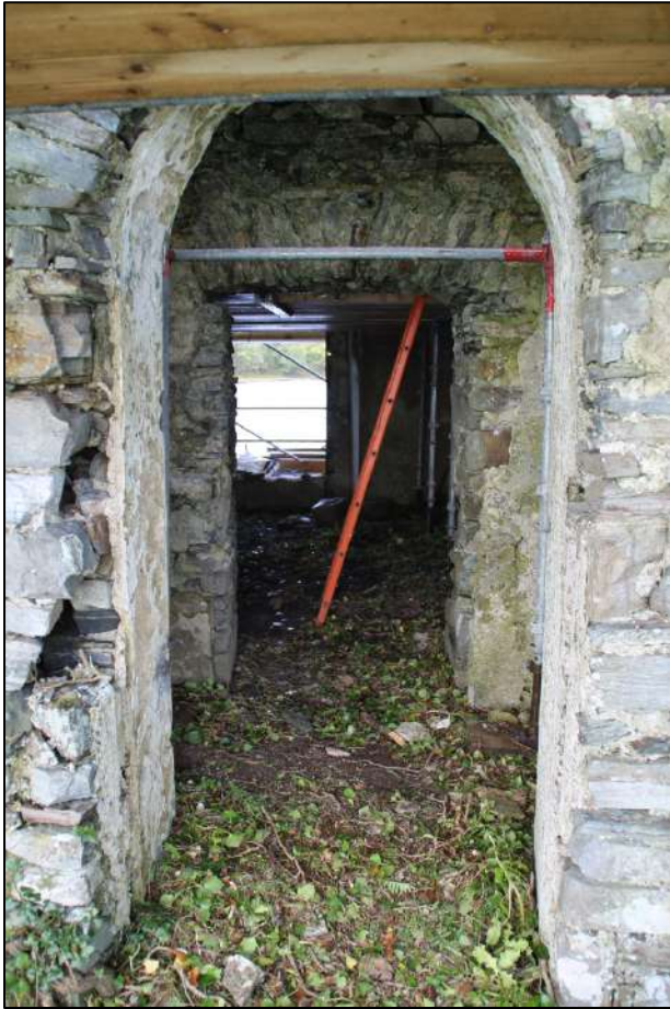
Pl. 2 Main entrance with doorway to ground floor chamber behind.
