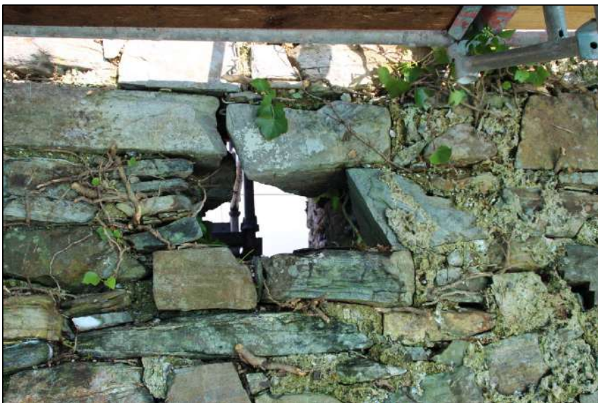
Pl. 38 This irregular opening belongs to a rectangular window high on the stairwell. It is larger internally.
