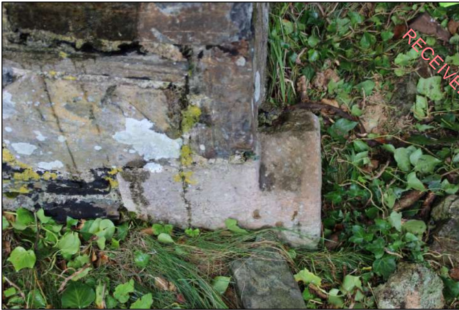
Pl. 110 Moulded door stop at base of large doorway on the northern wall.
