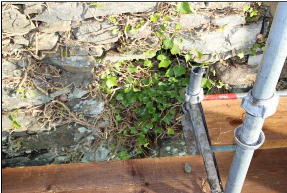
Pl. 42 Small irregular opening at second floor level, southern side of the tower house.
