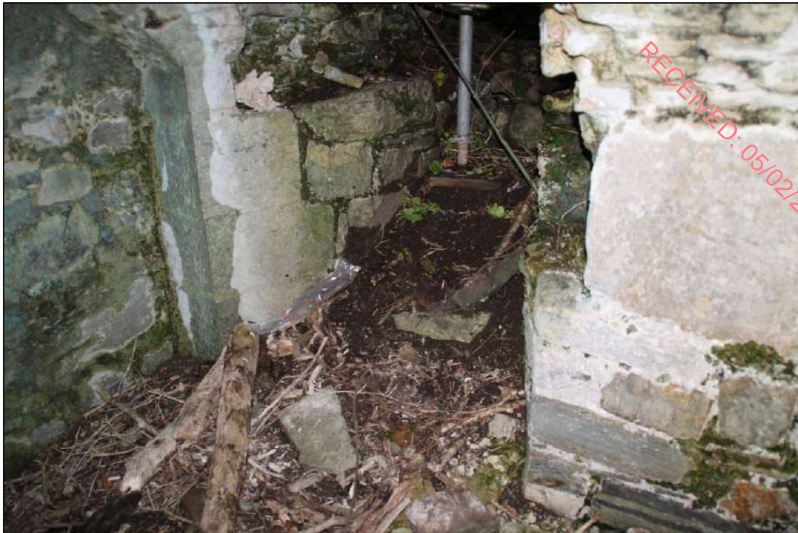
Pl. 141 The lower part of the drawing hole of kiln 2.
