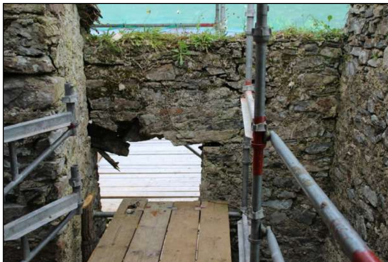
Pl. 78 The wall forming the north-east corner, a later construction now in poor repair
