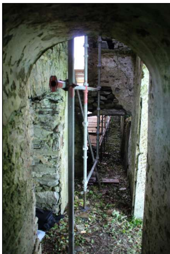
Pl. 43 The entrance lobby looking northwards.
