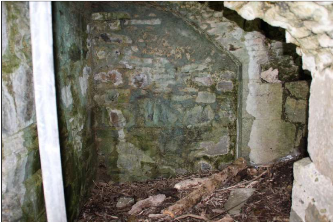
Pl. 138 The interior of kiln 2 looking east. The drawing hole of the kiln is on the right. This structure is a later addition to the industrial complex on the island.
