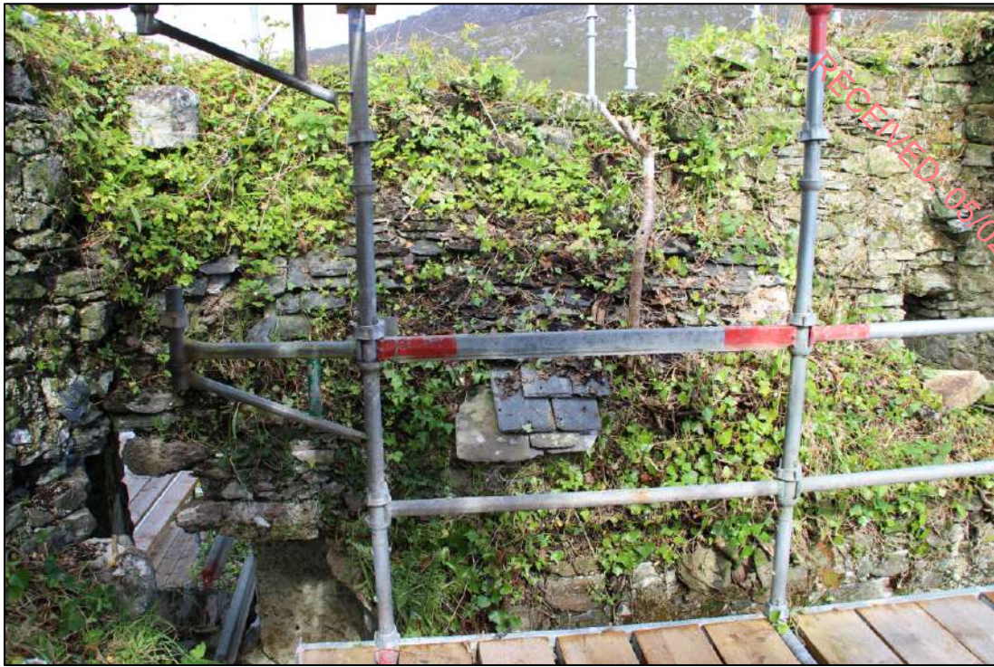
Pl. 100 The weatherslated panel in the north-western corner of the second floor. This is laid sloping towards the interior of the building. The opening in the masonry on the left exposes the 'oriel' chamber.
