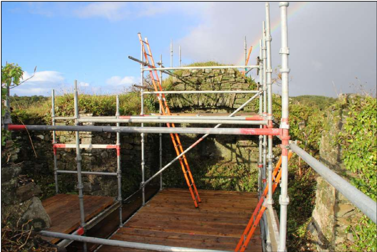
Pl. 95 The second floor of the tower house looking west.
