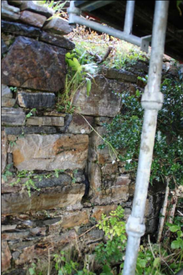
Pl. 113 The slit window on the western side of the large room of the industrial building.
