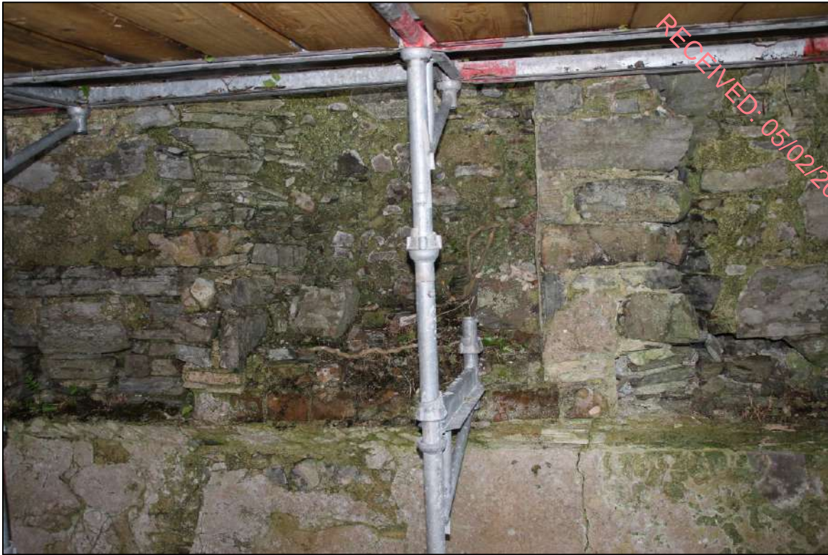
Pl. 82 Base of fireplace. Note the bricks in the base of the hearth.
