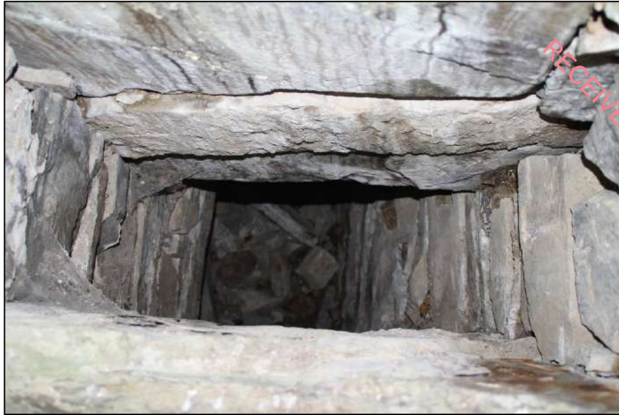
Pl. 70 View down the garderobe shaft. There is no evidence of an exit chute.
