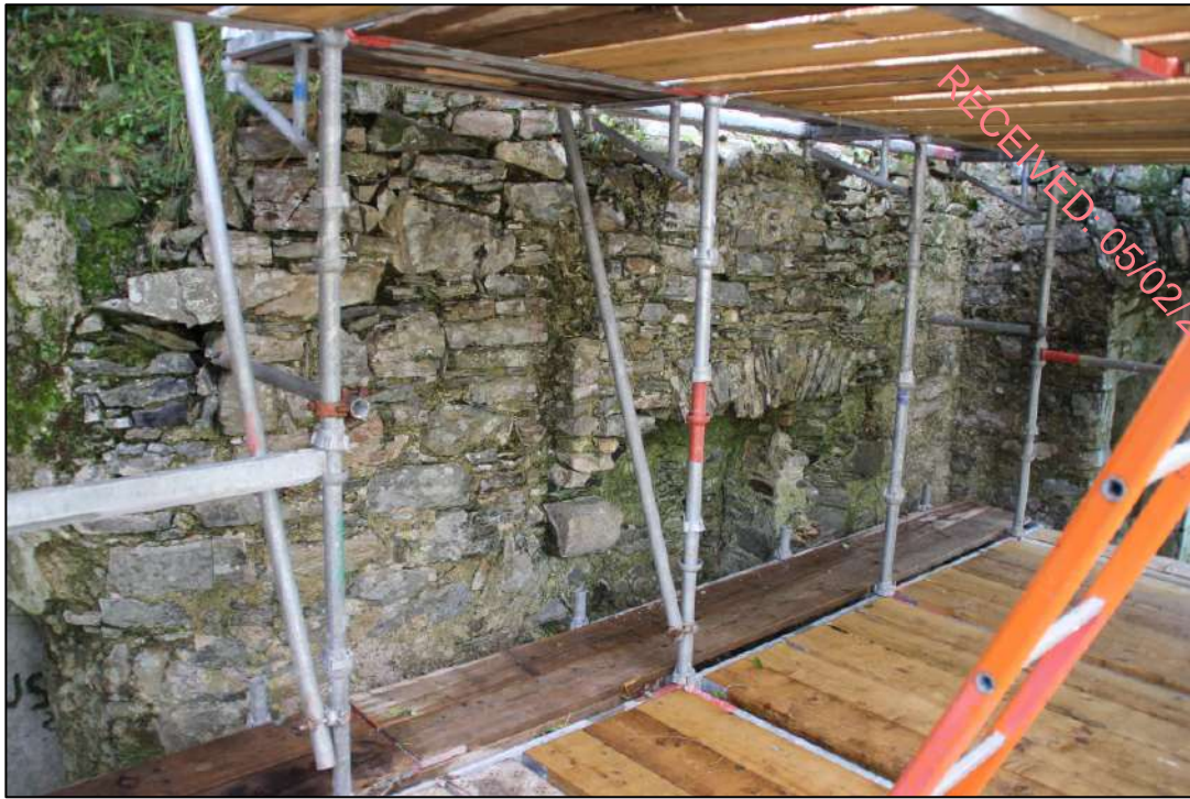
Pl. 80 The southern wall of the first floor.
