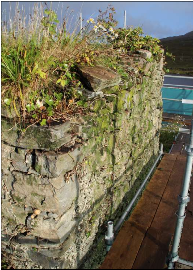
Pl. 1 Top of tower house, eastern side.
