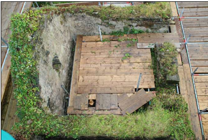
PI. 143 The chimney in the south-eastern corner of kiln 2. This is built of handmade brick.
