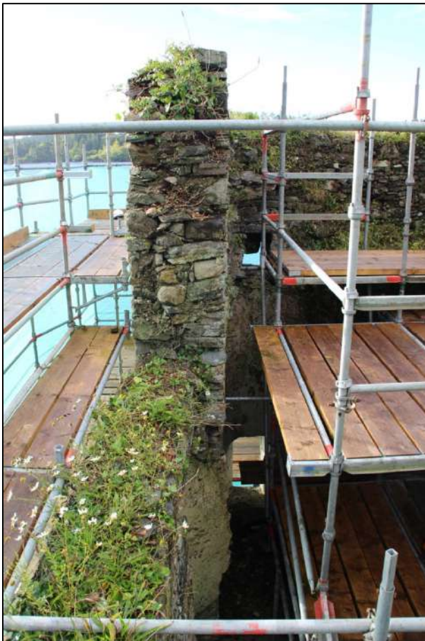
Pl. 11 Unusual bedding of stones may mark a blocked ope on the upper part of the stairs.
