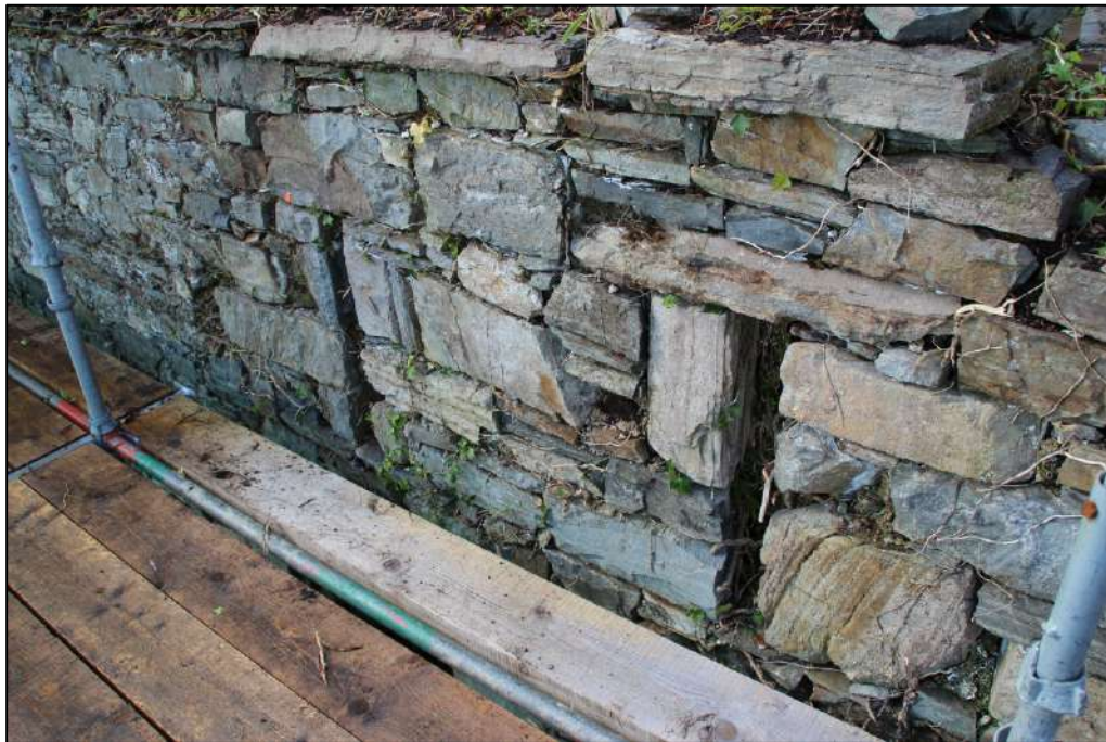
Pl. 108 Slit openings in the central part of the first floor of the industrial building. Note the two cornice stones.
