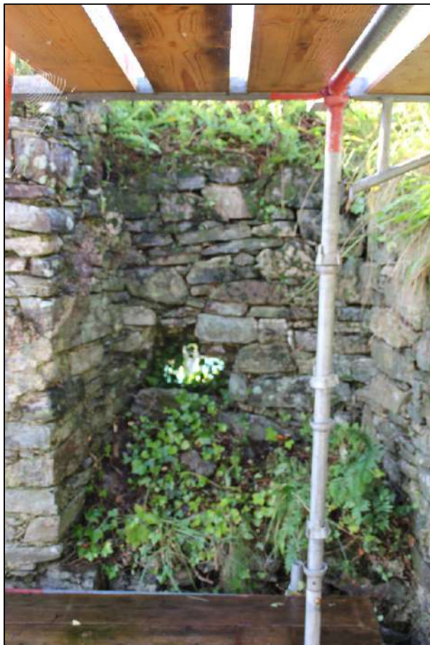
Pl. 100 The weatherslated panel in the north-western corner of the second floor. This is laid sloping towards the interior of the building. The opening in the masonry on the left exposes the 'oriel' chamber.
