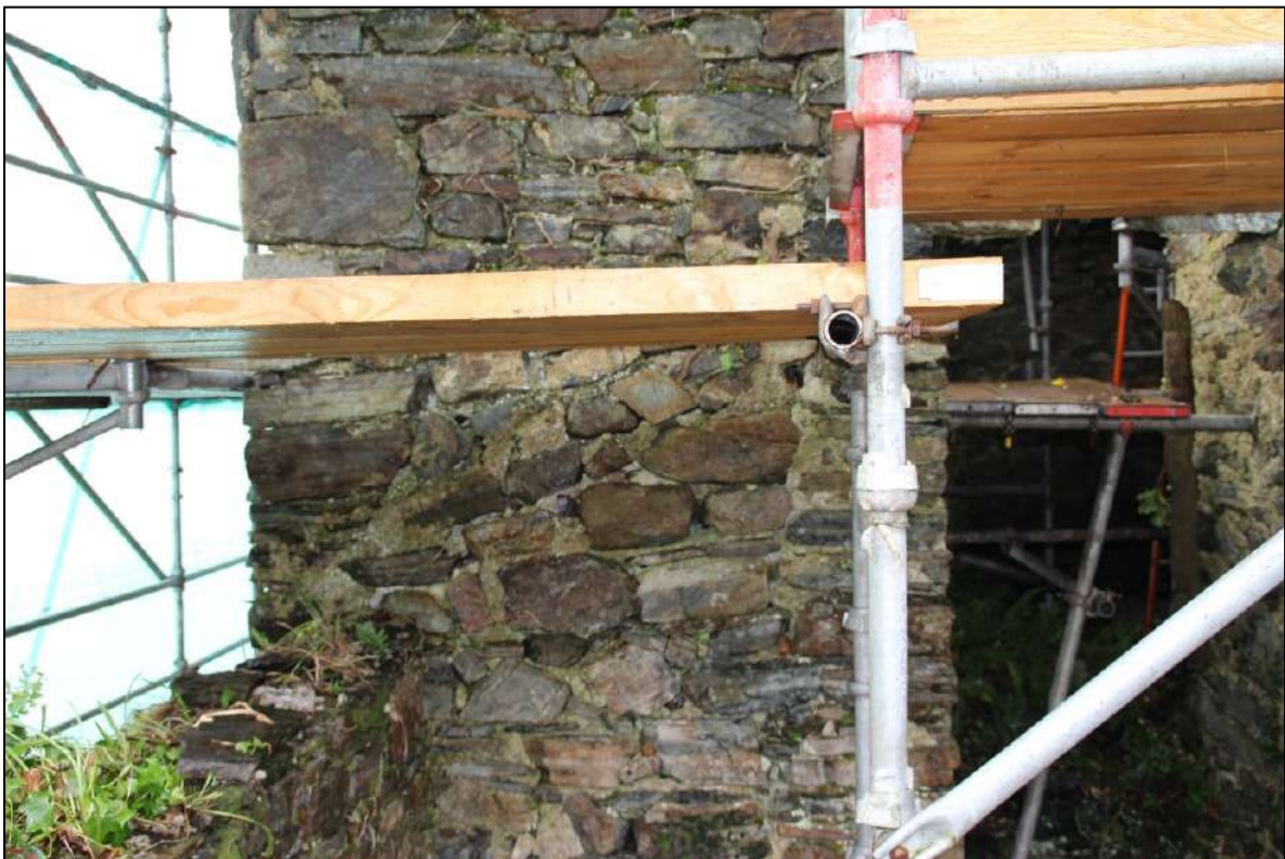
Pl. 146 Mortar scar evident running from the top of the wall on the left towards the top set of scaffolding planks. This marks the position of the roof over the large room of the industrial building.
