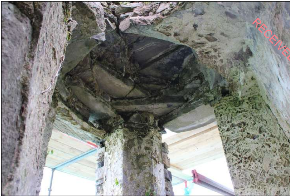
Pl. 92 The corbelled roof of the 'oriel' chamber.
