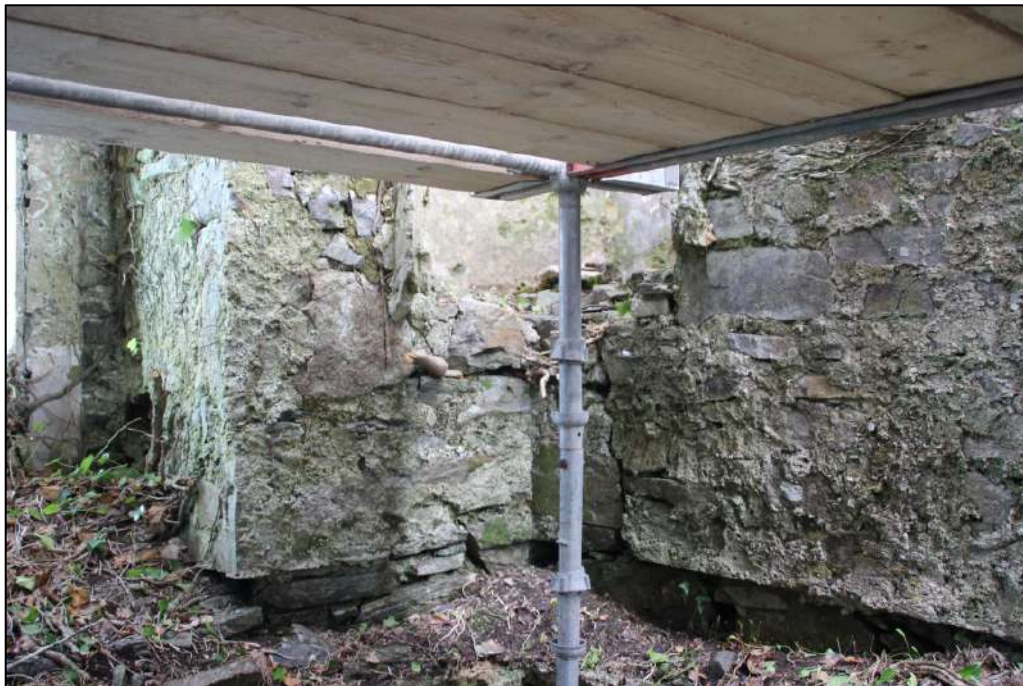
Pl. 89 The difference in levels between the floor of the main chamber, represented by the linear scar in the masonry and the higher level of the 'oriel' chamber floor.
