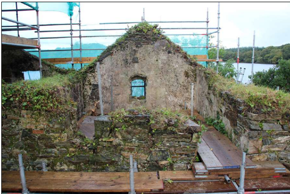
Pl. 142 The first floor room over kiln 2. The doorway is on the right. Like in the first floor room of kiln 1, this is also plastered internally.
