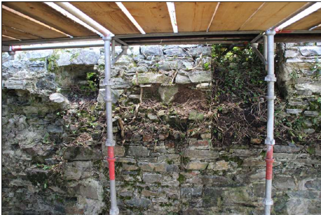
Pl. 127 The large opening on the upper right is the doorway leading to the room over kiln 2. On the upper left is a small opening (vent?) into the same area. The fireplace can be seen in the lower left. The vertical break in the masonry in the bottom centre of the photograph may be the remains of a (slit?) window that was blocked when kiln 2 was constructed.
