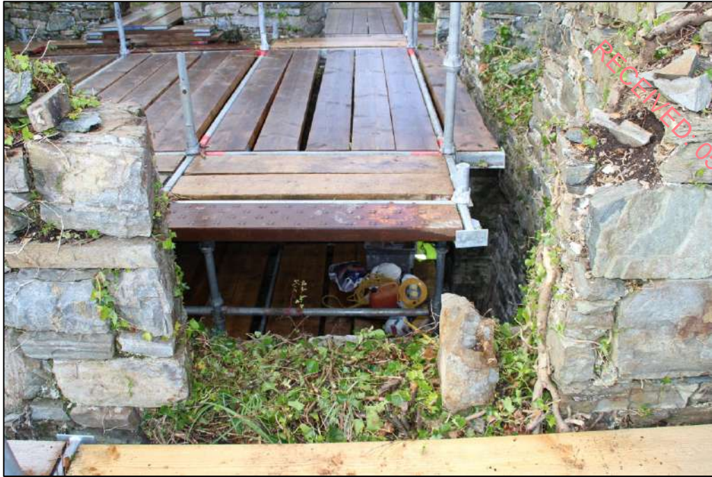
Pl. 107 The larger window at the northern end of the first floor of the building, eastern elevation.
