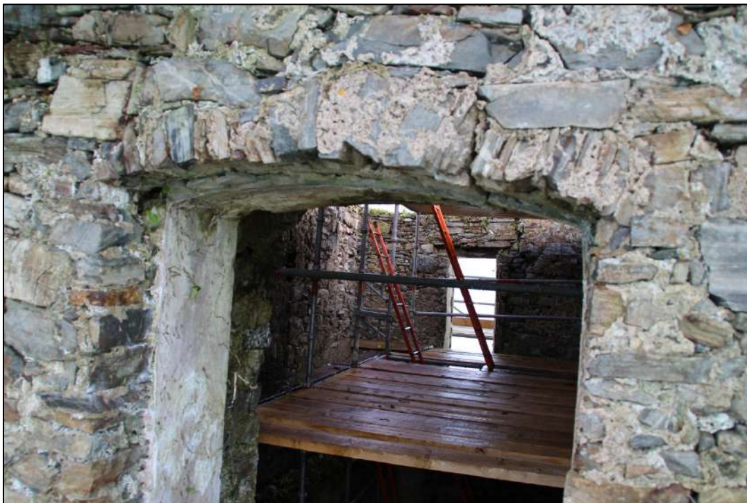
Pl. 22 The head of the large window on the western side of the first floor. This later held a wooden sash window.
