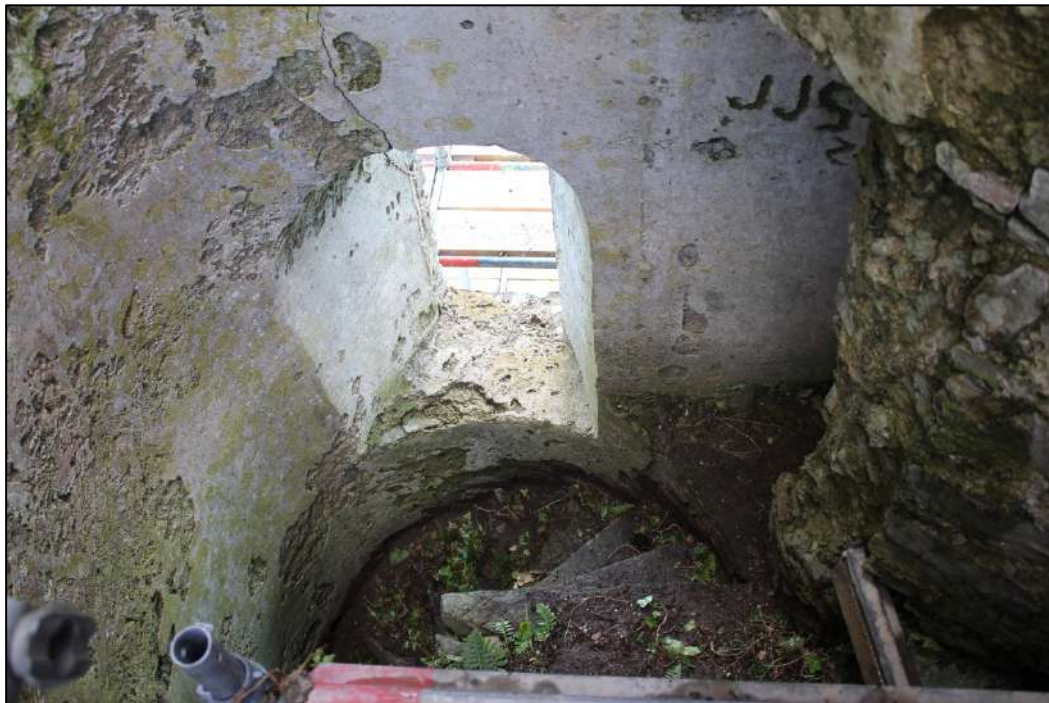
Pl. 61 View of the stairs, the splayed window opening, the garderobe passageway (on centre right) and the entrance to the main room of the first floor (on lower right).
