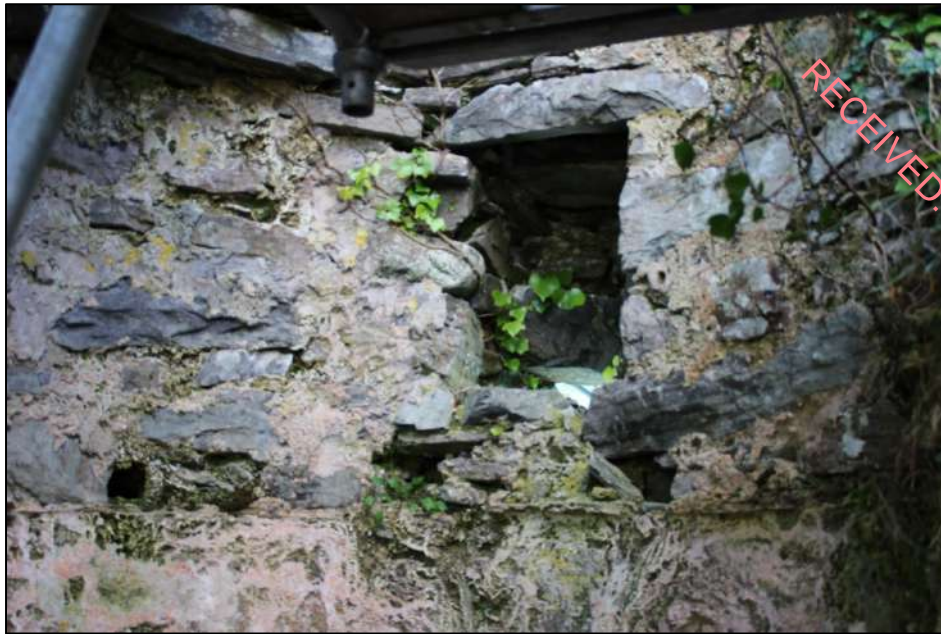
Pl. 66 Detail of the opening and the ceiling supports. This window is much smaller on the outer face of the wall.
