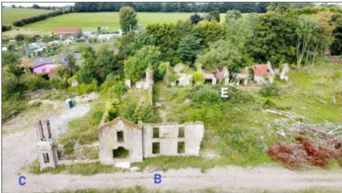
Figure 3. Aerial view of site buildings B - old hydropathic facility; C – Belfry; E Stables and Coach house (with corrugated roof at right of photo)
