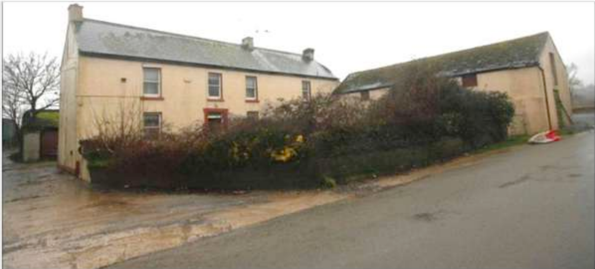
Plate 1. Farmhouse (on left) and Building B adjoining outhouse (on right) to be refurbished for housing
