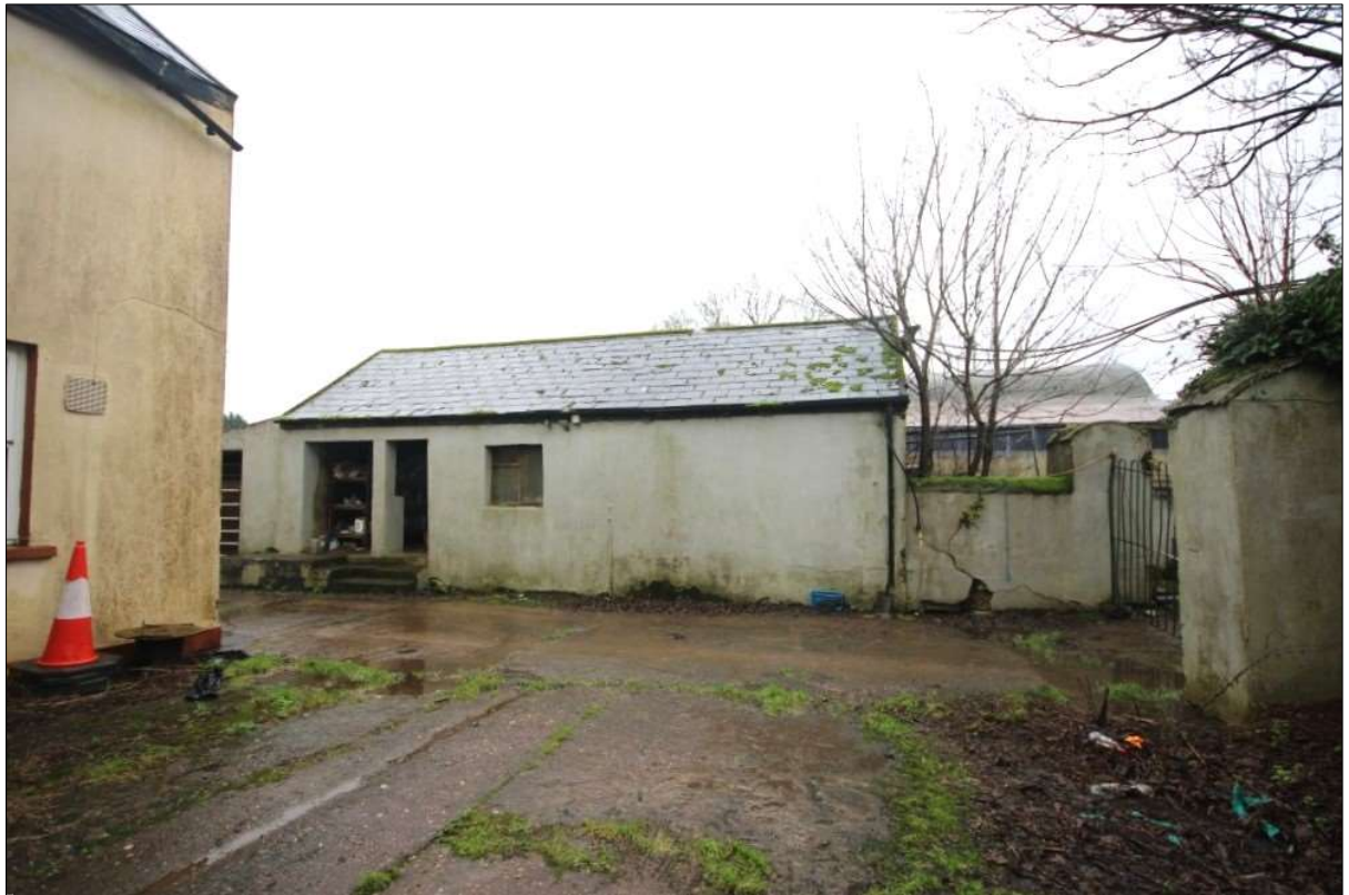
Plate 58: Northern elevation of outbuilding Building D. Note this shed to be demolished .
