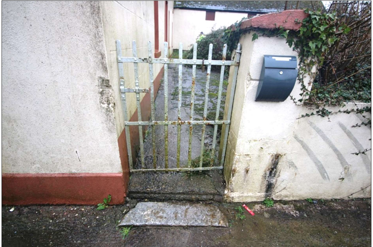
Plate 8: Wrought iron pedestrian gateway to be retained.
