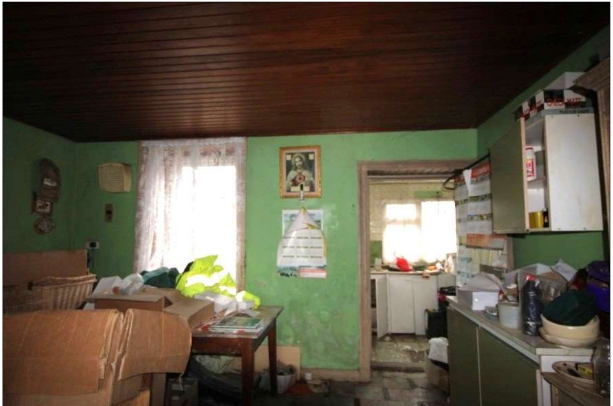
Plate 19: Kitchen A-GF05 looking to rear. Scullery to distance . Note cement rendered kitchen walls painted green and modern timber sheeted ceilings
