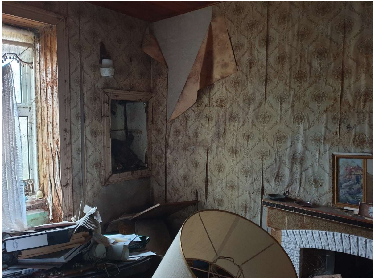
Plate 38: Detail of Niche to Tv room
