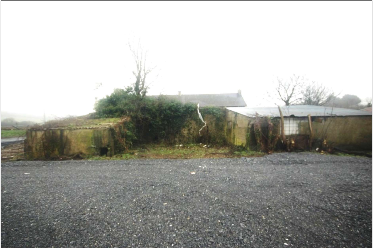
Plate 4: Rear elevation of outbuildings to west
