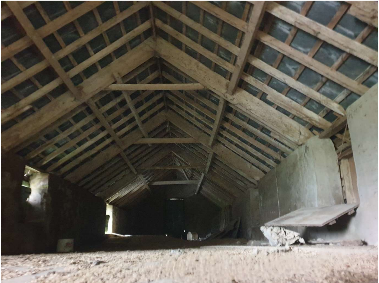
Plate 51: Building B -Barn – View of first floor structure, inaccessible for surveying.
