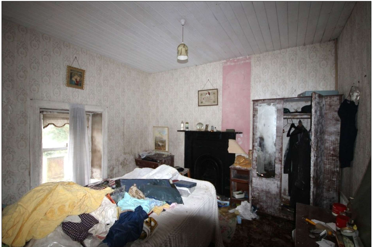
Plate 30: First-floor bedroom facing west to rear off landing AFF05.
