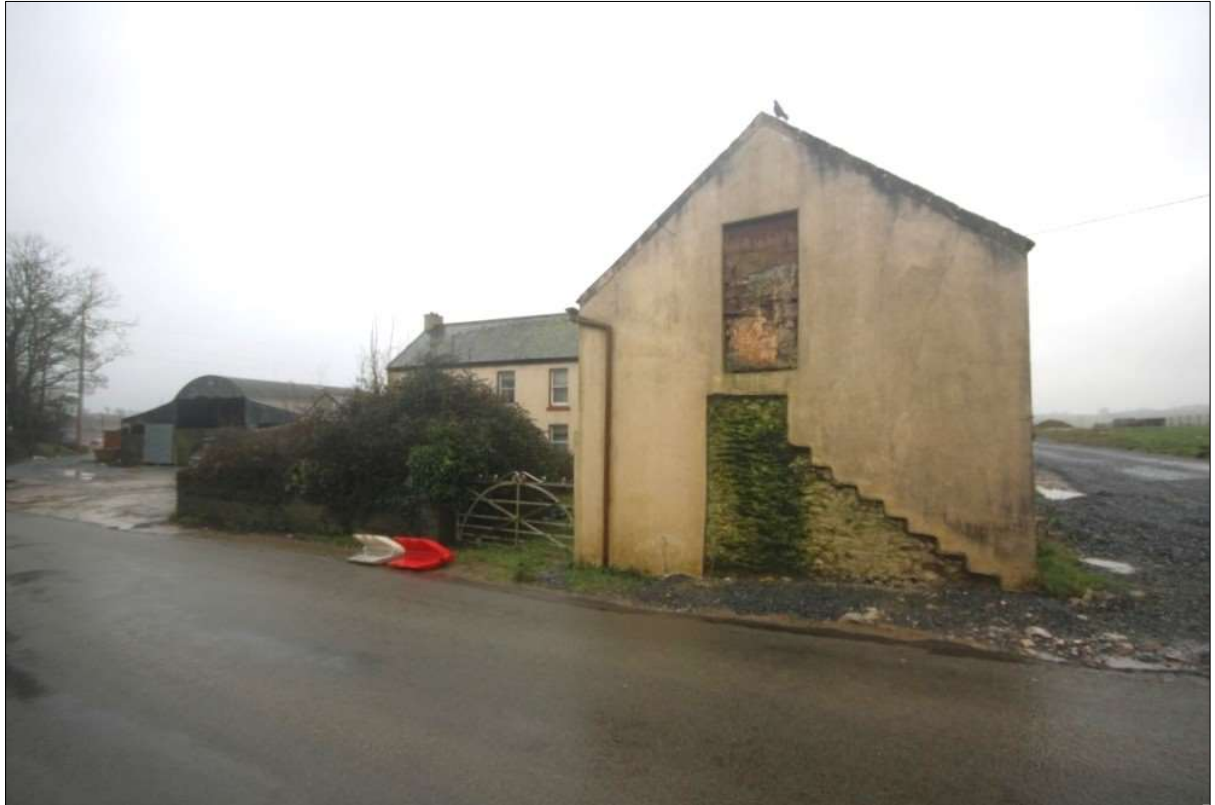
Plate 45: Eastern elevation of Building B-Barn. Note steps are no longer extant. Note limestone wall coursing to exposed render.
