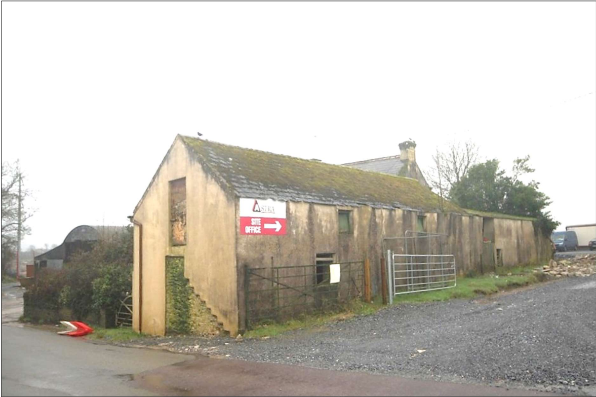
Plate 2: General view to subject site looking southwest
