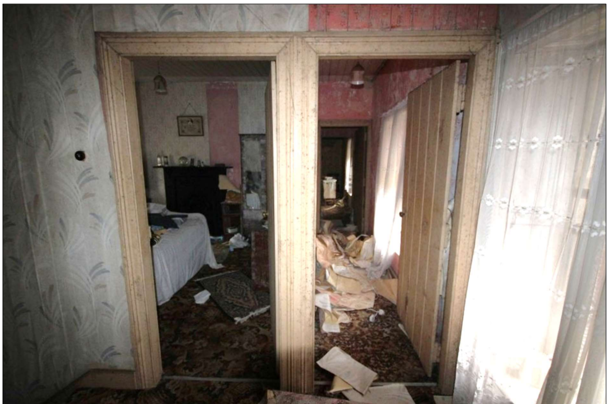
Plate 25: Doorways to Bedrooms A-FF02 and AFF05 on main landing. Note short lobbied corridor to RHS similar to ground floor arrangement. Architraves and doors appear original .
