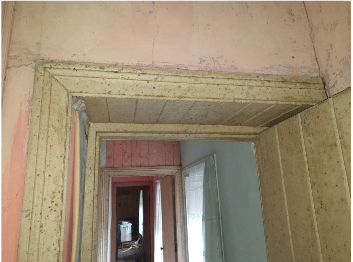
Plate 34: Detail of moulding to room AFF07
