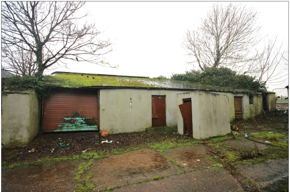
Plate 54: Eastern elevation of outbuilding Building C. This space is to be converted to an apartment.
