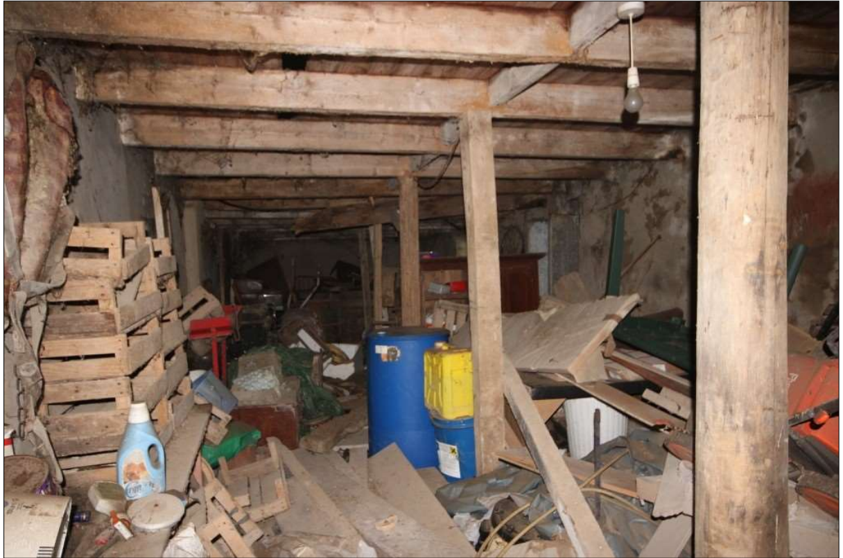
Plate 49: Ground floor Building B. Note reinforcing props.
