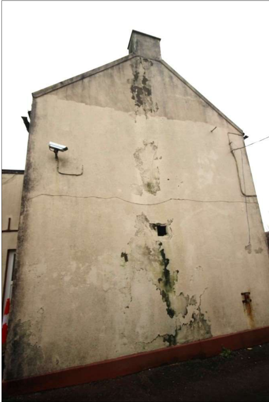
Plate 6: Southern elevation of Building A Main house gable
