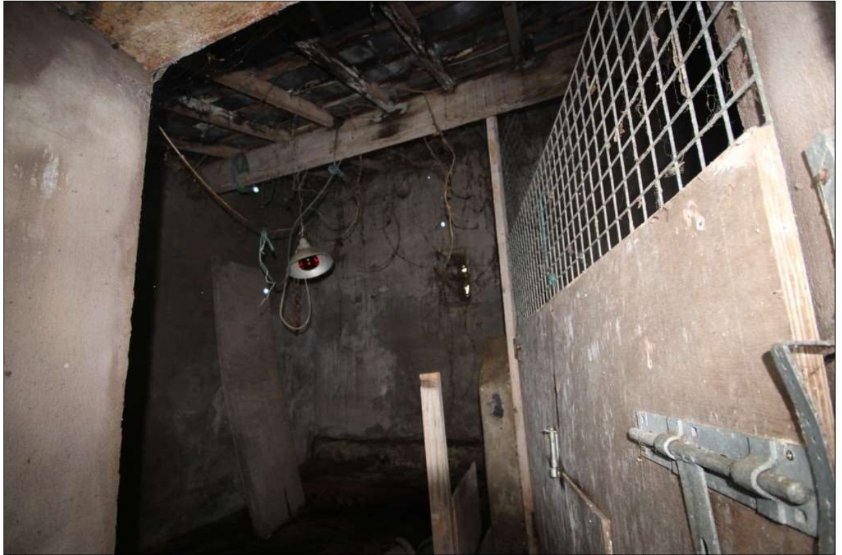
Plate 55: Interior of outbuilding Building C
