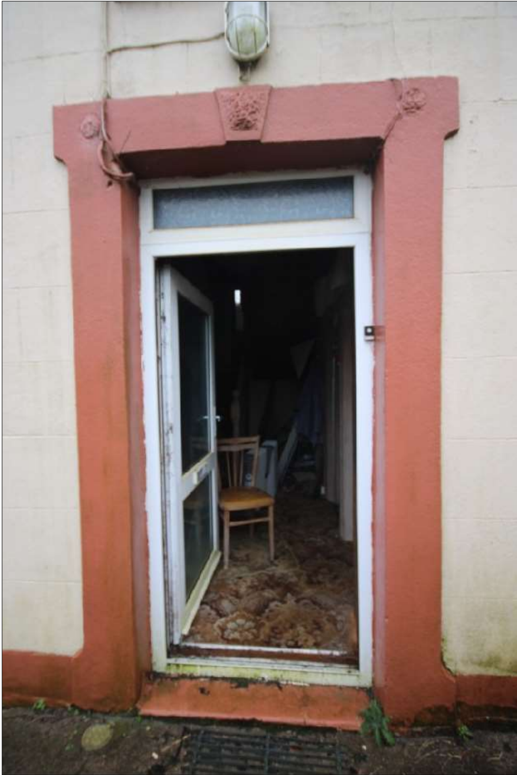
Plate 12: Replacement aluminium front door with rendered detail to be retained.
