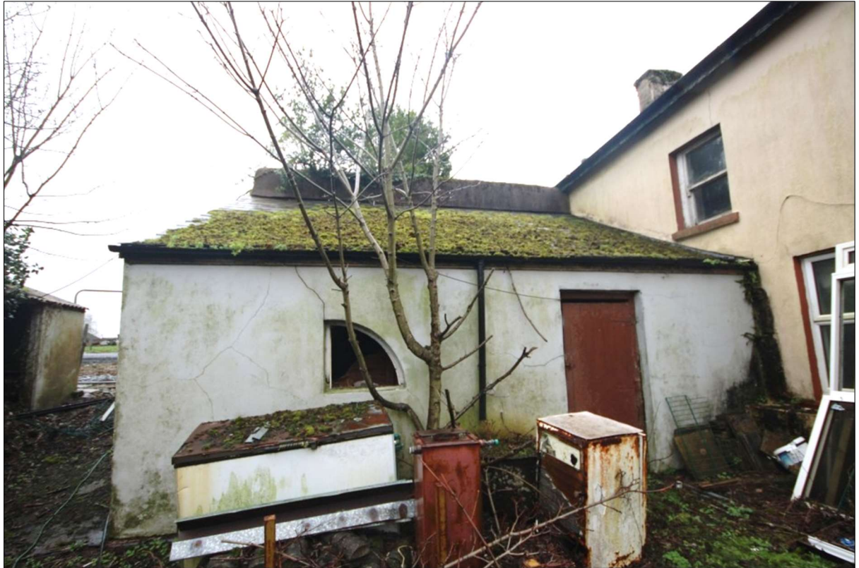
Plate 52: Single-storey return to Building A. This annex may be contemporary with the main house and the barn behind added and adjusted subsequently
