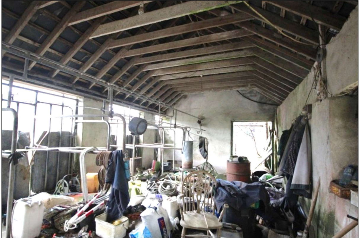
Plate 60: Interior of Building D. Note this shed is to be demolished .
