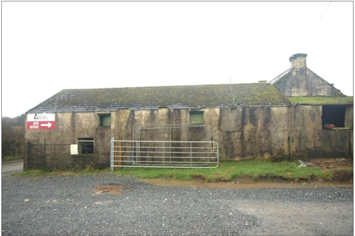
Plate 46: Northern elevation of Building B-Barn. Note slates here appear artificial and may contain asbestos.
