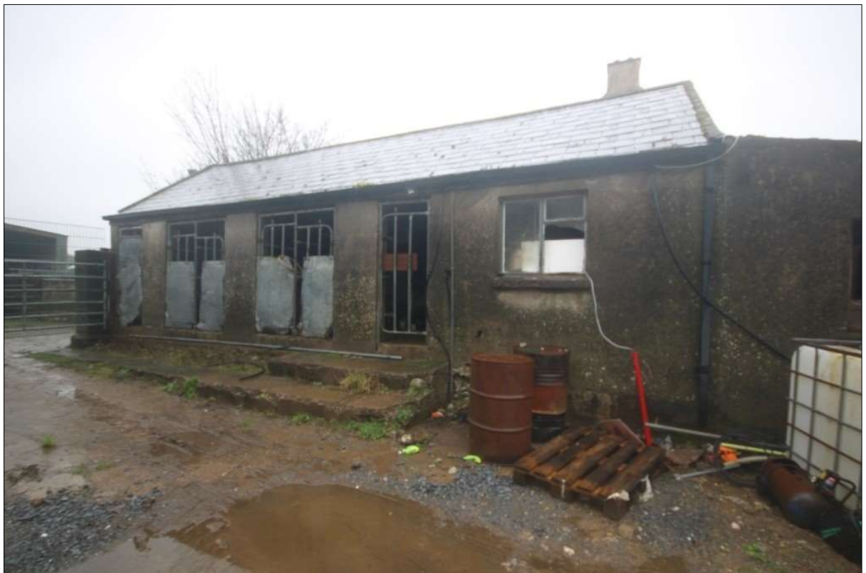
Plate 59: Southern elevation of Building D. Note this shed is to be demolished.
