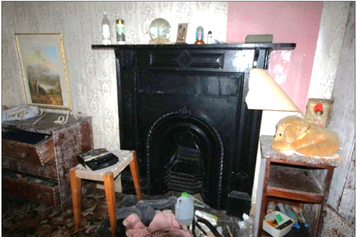
Plate 31: Cast iron fireplace in A-FF05
