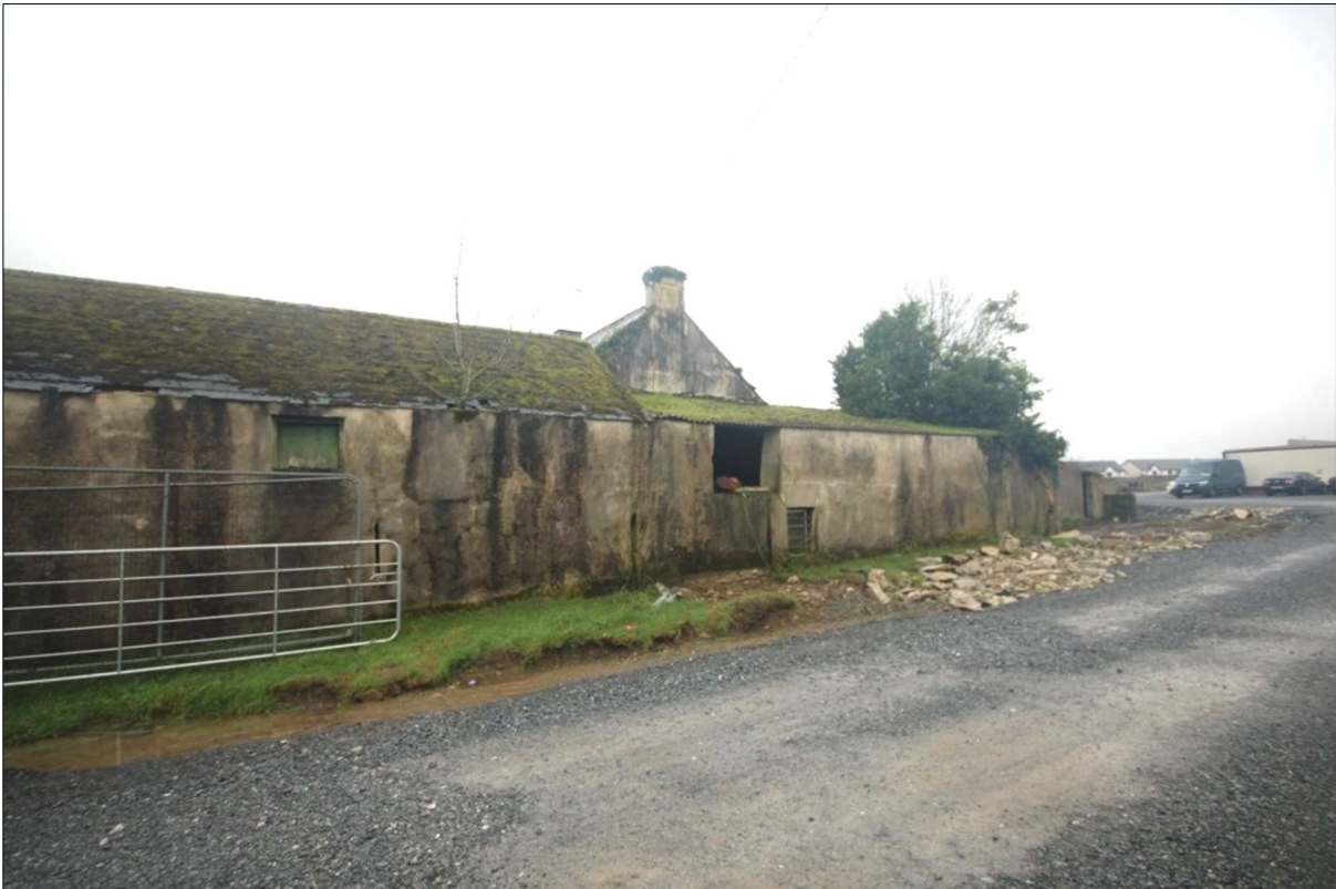
Plate 3: Northern elevation of outbuilding, Building B-Barn
