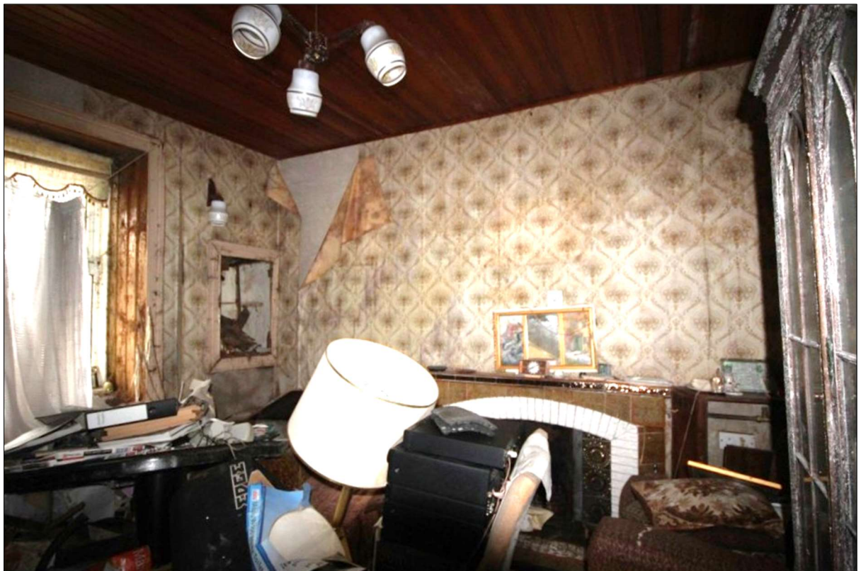
Plate 17: Ground floor Tv room A-GF04. Note marble tile fireplace , Niche to corner and modern timber sheeted ceiling.
