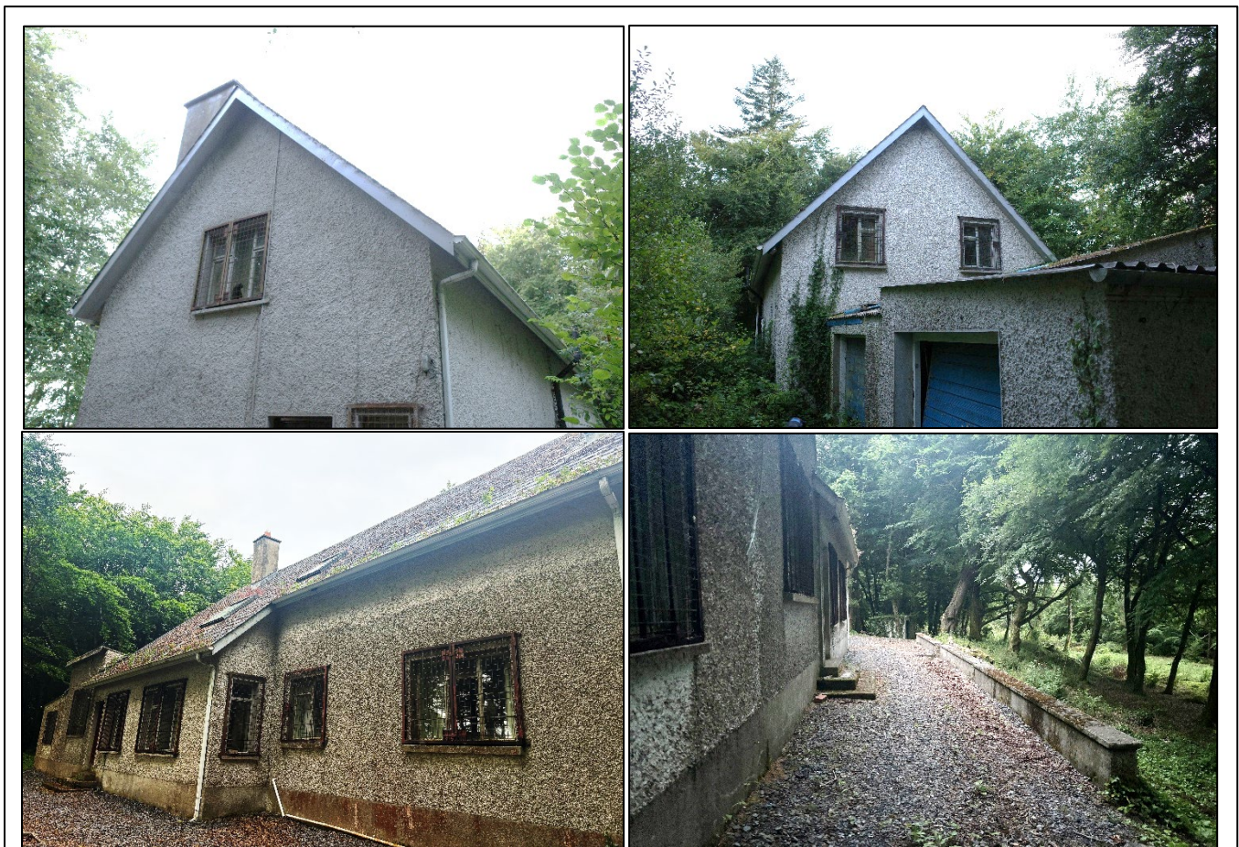
Plate 3.1: Survey Observation Points for Emergence and Re-entry of building
