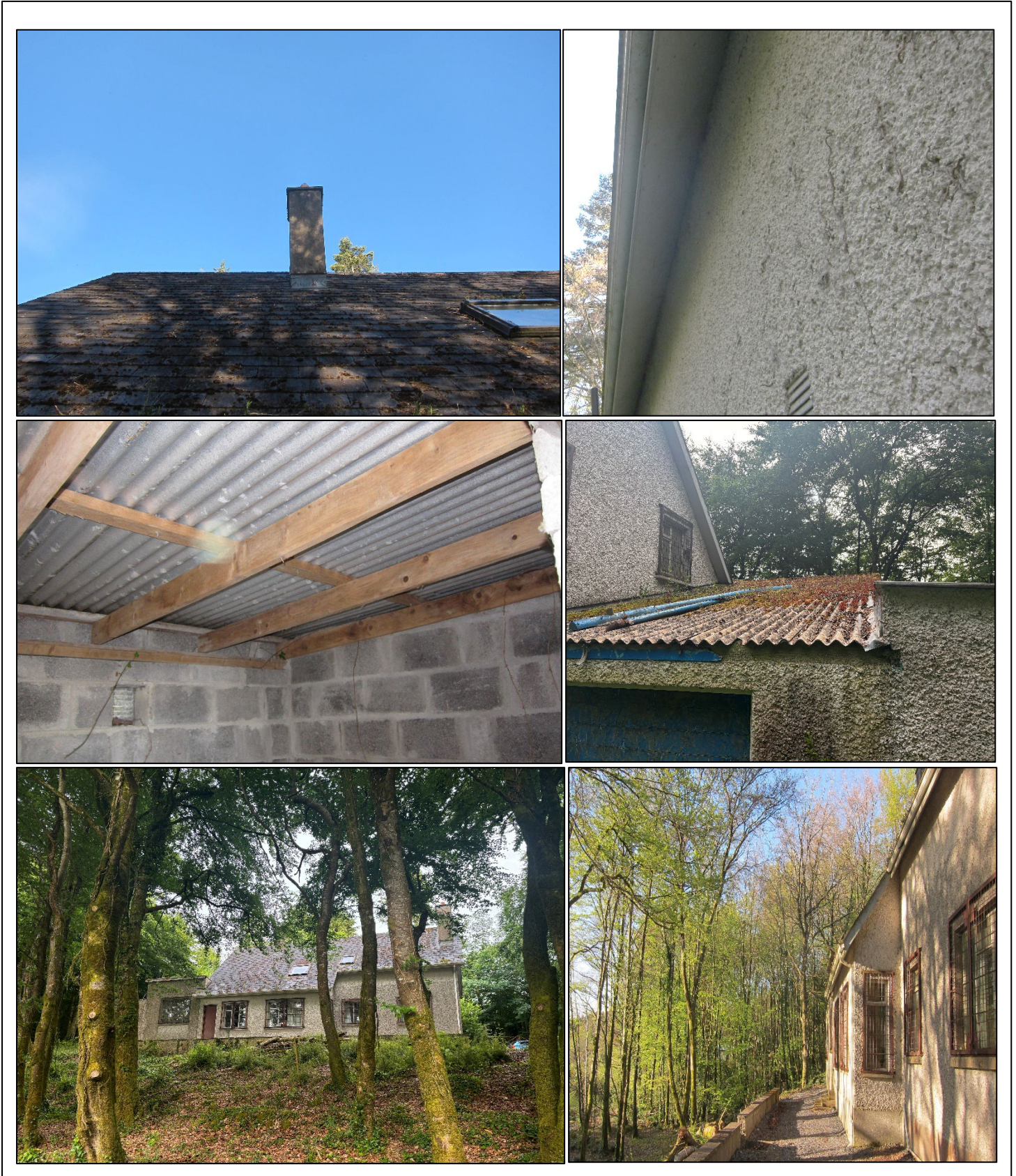
Plate 4.5: Assessment of house, garage, outbuildings and surrounding site
