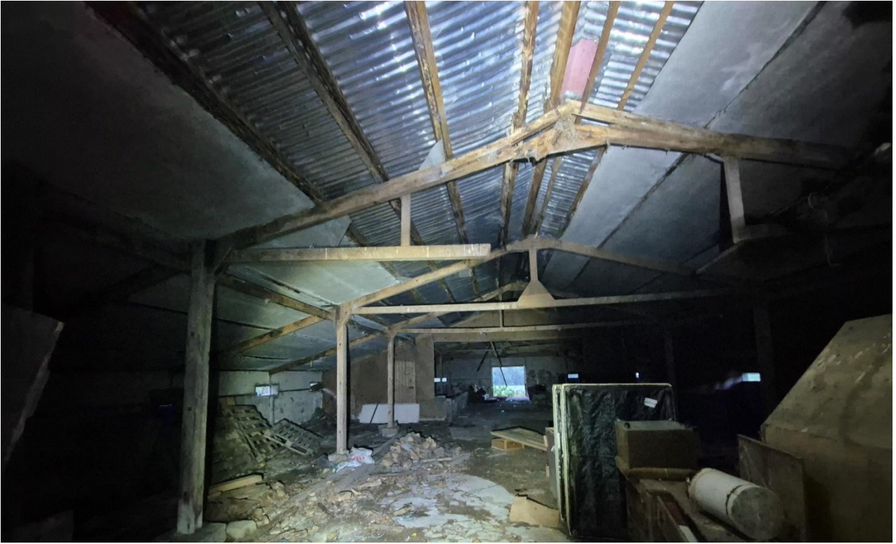
Plate 3: Internal photograph of Shed A (Building 3), Cornacassa, Monaghan Town, Co. Monaghan.
