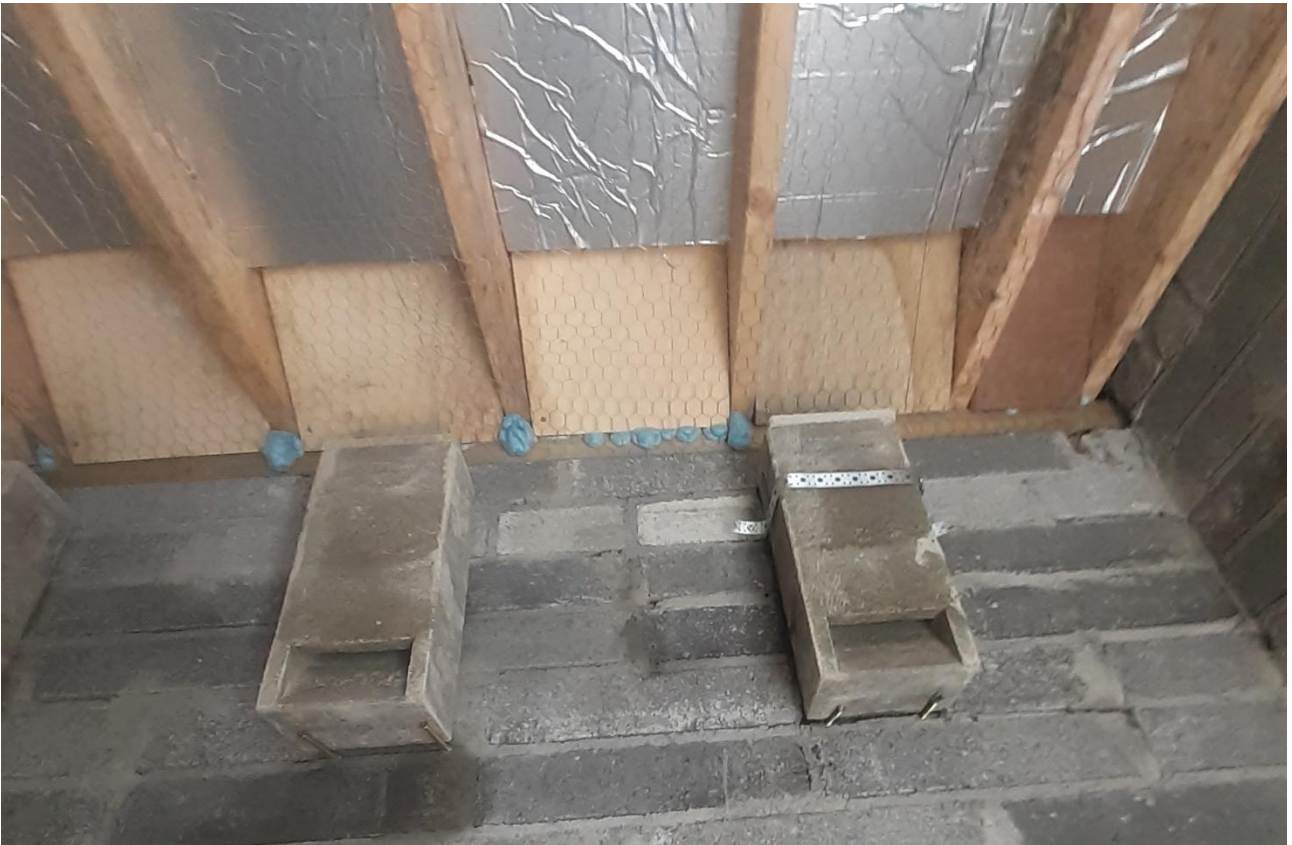
Bat Tubes fixed onto internal ground floor wall (Oldstreet Substation bat House, Co. Galway).
