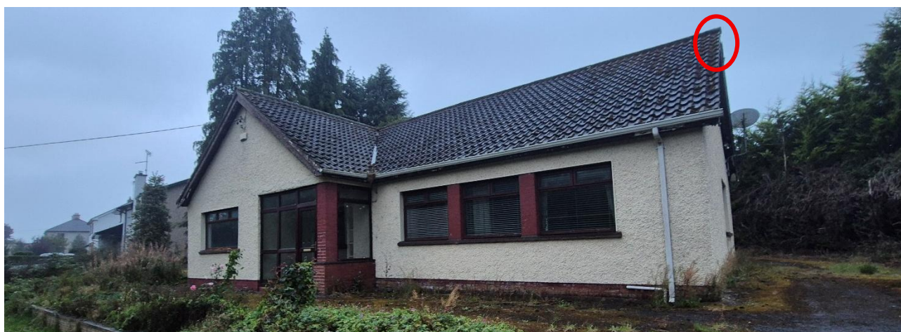
Plate 6: Exit point for brown long-eared bats from roof space of bungalow (Red circle).
