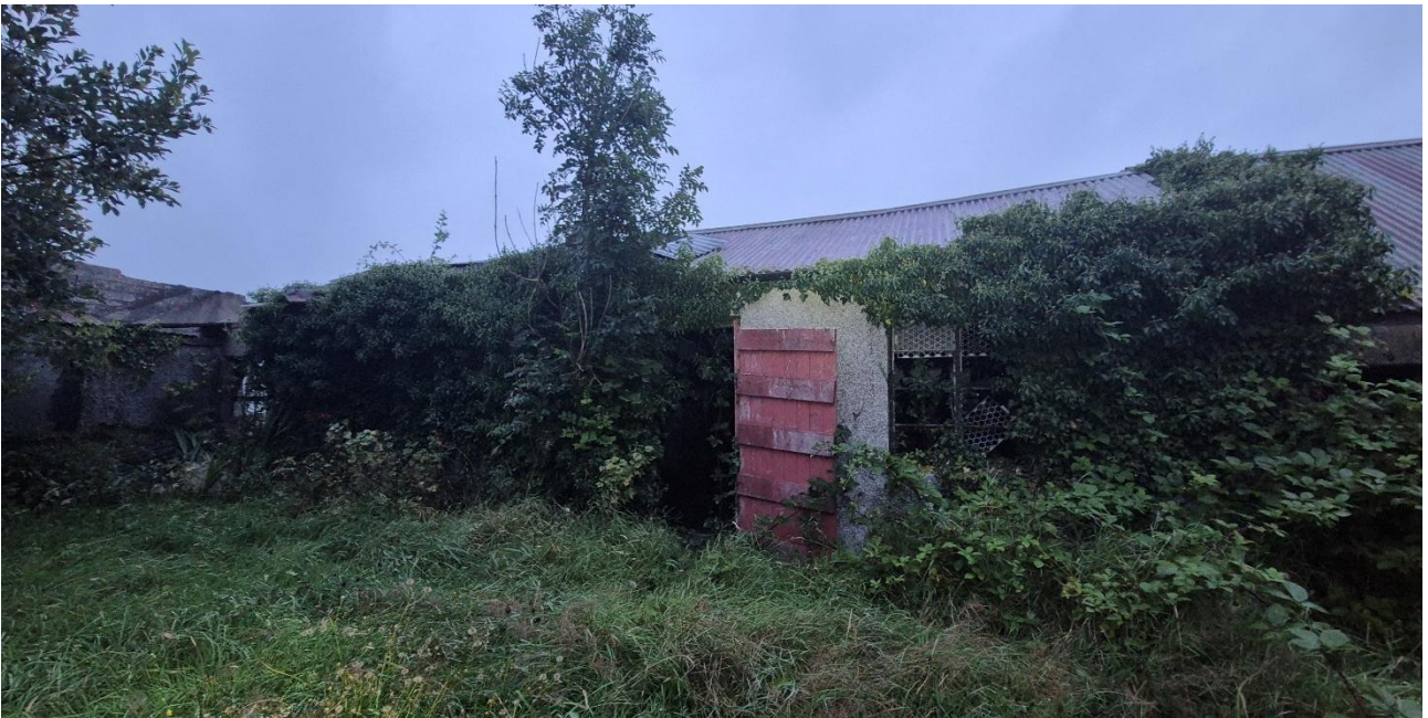
Plate 4: External photograph of Shed C (Building 5), Cornacassa, Monaghan Town, Co. Monaghan.
