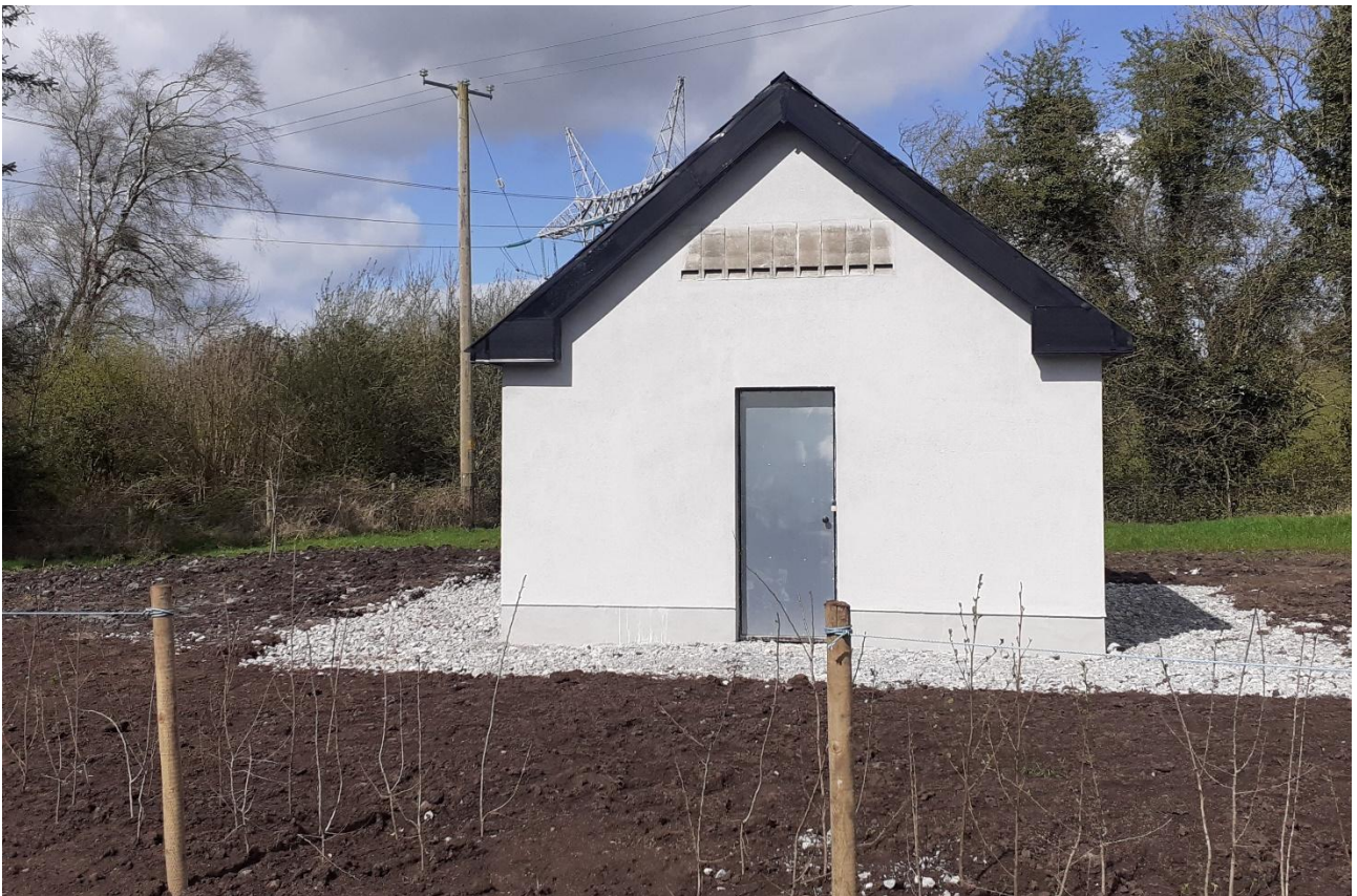
Finished bat house with bat tubes (south facing external wall), Oldstreet Substation Bat House, Co. Galway.
