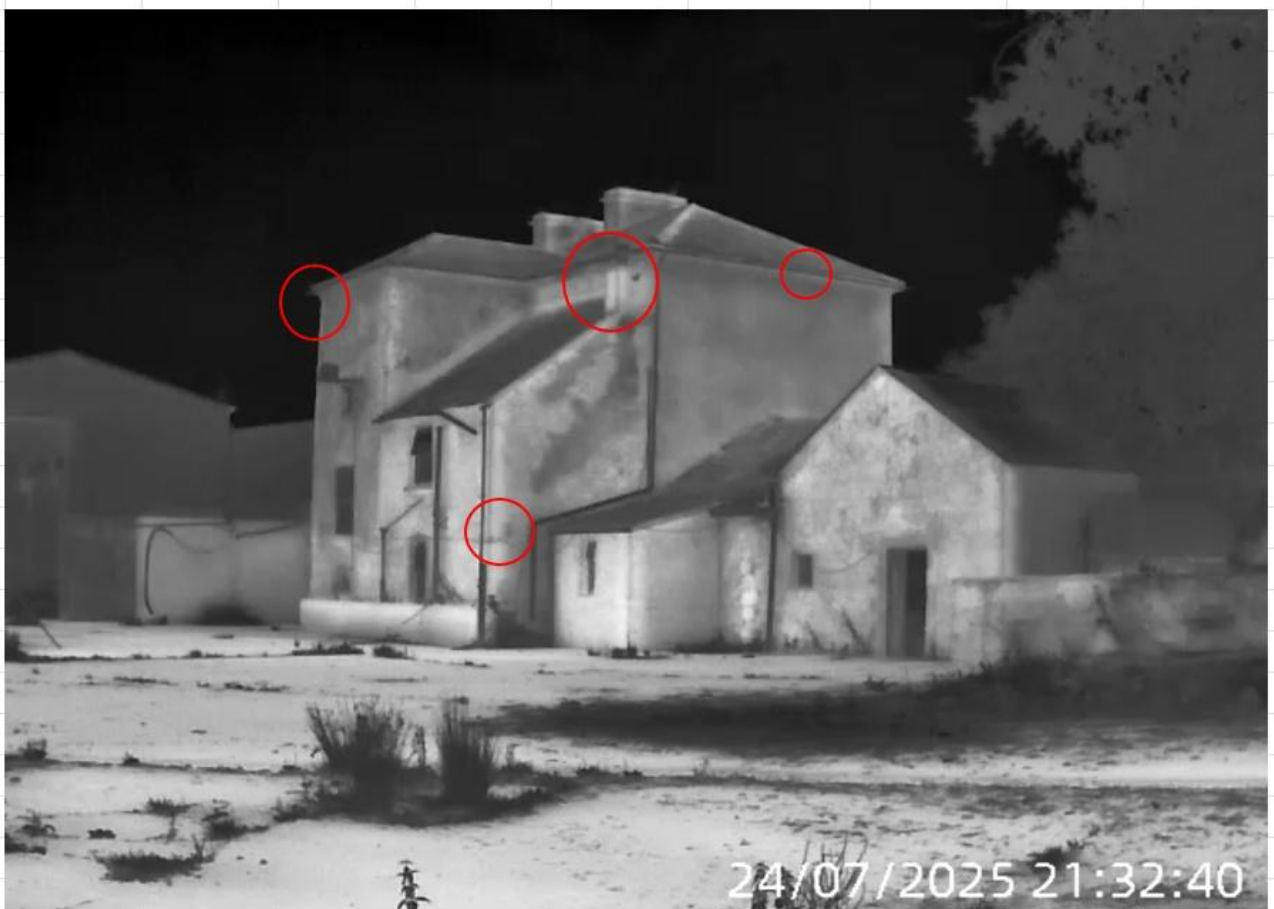
Plate 8-3: Exit points to rear of existing residential building
