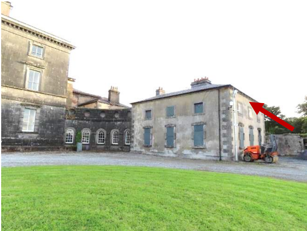
Figure 9: Western wing of Hazelwood House, and location of the Soprano Pipistrelle roost
