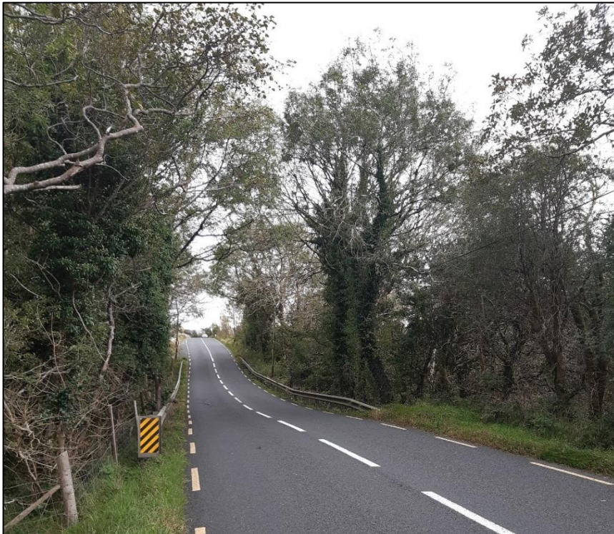
Figure 2.1 Glenmore Bridge with narrow cross section and poor vertical alignment
