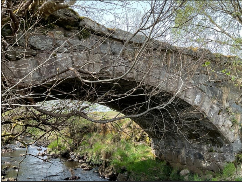
Figure 2.2 South side of Rive Derg railway bridge.
