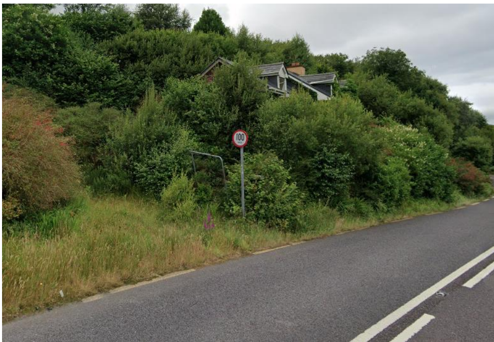
Plate 2 – Photograph of Griffins Cottage July 2023 – view west from N70
