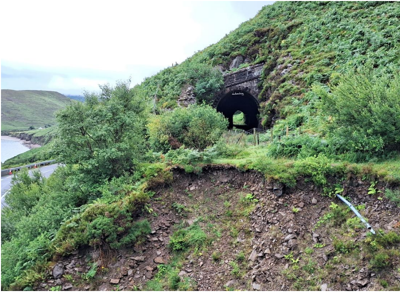
Plate 3 – Photograph of Drung Hill Tunnels (view east to middle tunnel).
