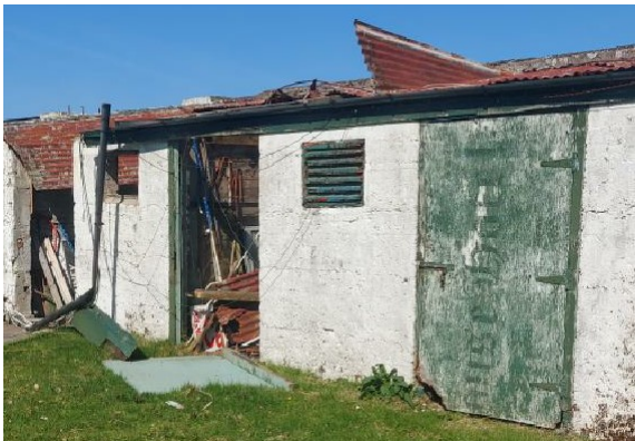
Plate 6. Roof damaged and partially missing
