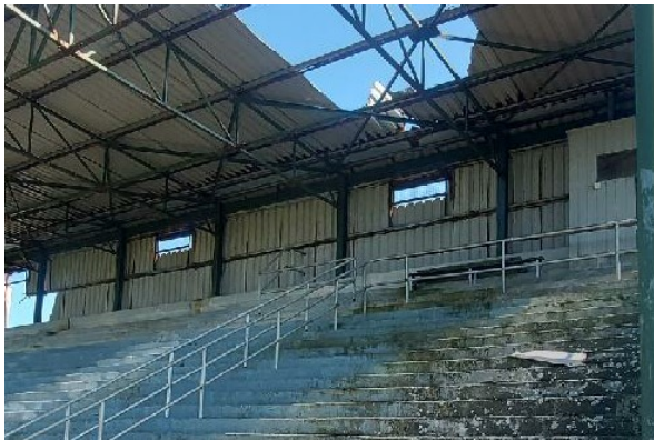
Plate 5. Roof damaged and partially missing
