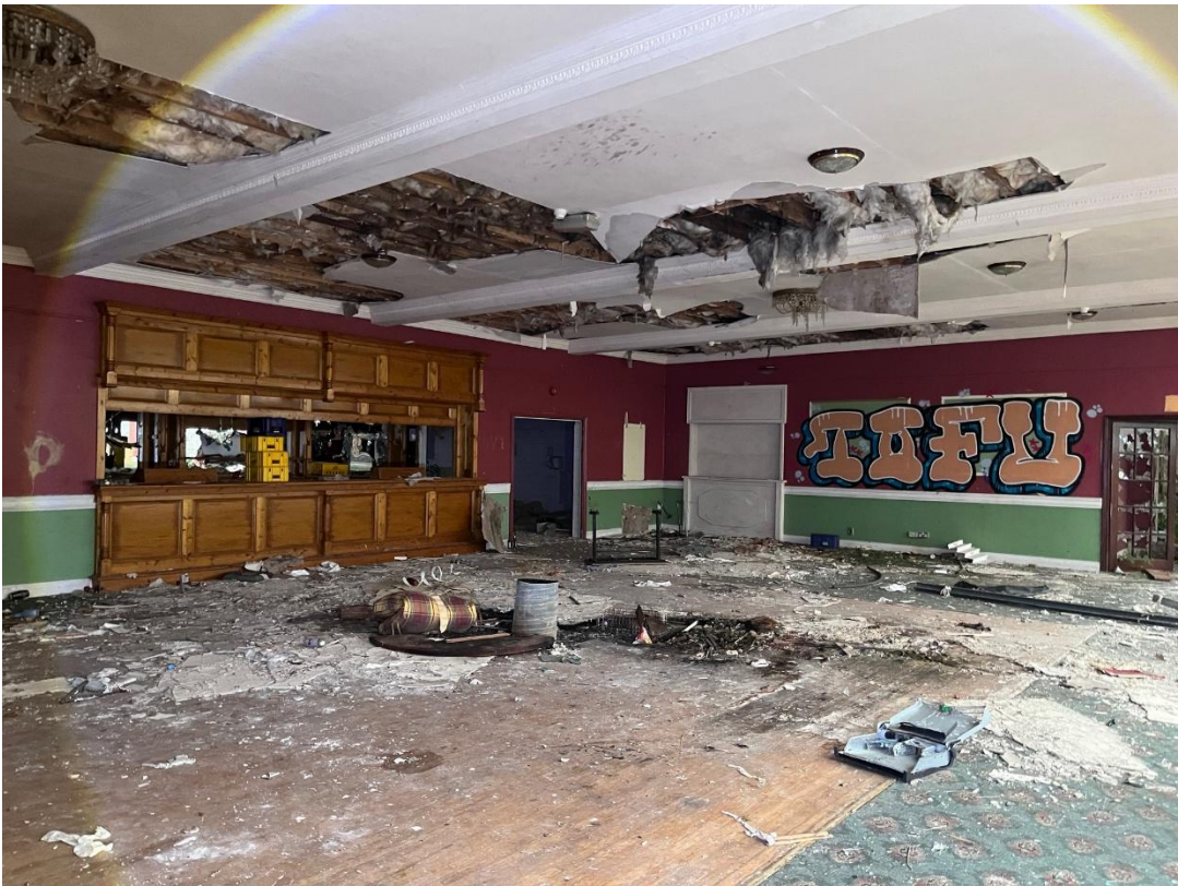
Plate 2 Photograph of internal room within hotel.
