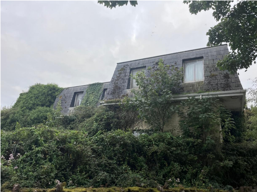
Plate 8 Northwestern end of hotel, photograph taken facing south.
