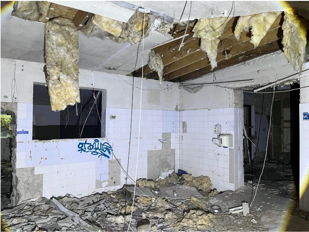
Plate 3 Photograph of internal room within hotel.
