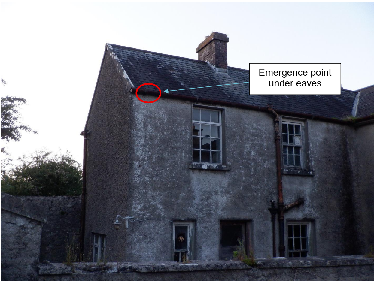
Figure 4-4: Rear of Garda station, showing bat emergence point.
