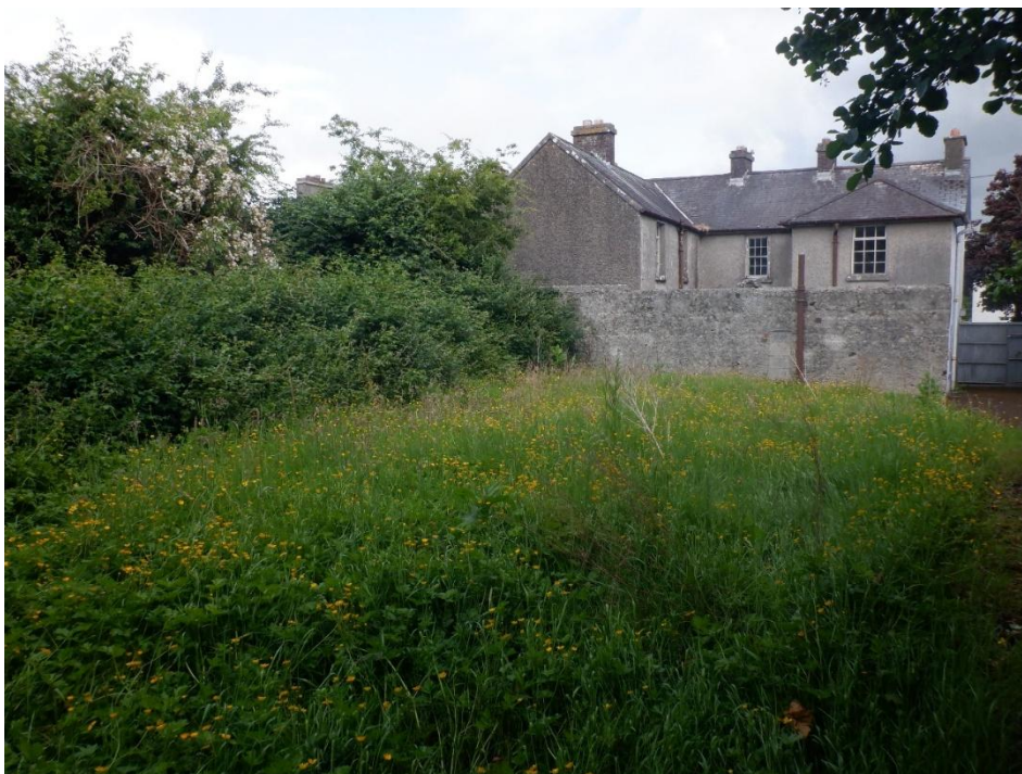
Figure 3-1: Rear view of garda station and adjoining garden.
