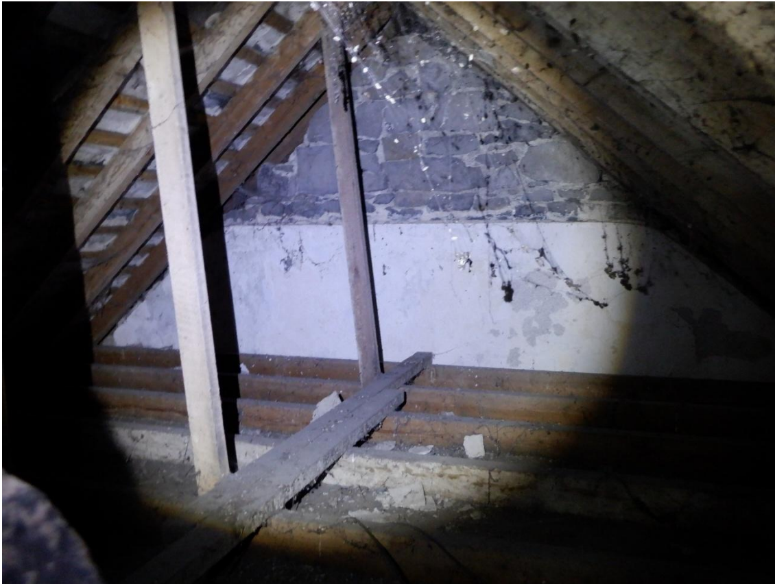
Figure 4-3: Wall in attic space in the central part.
