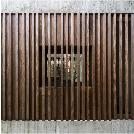
Figure 5-1: Example of louvred window to reduce light spill
