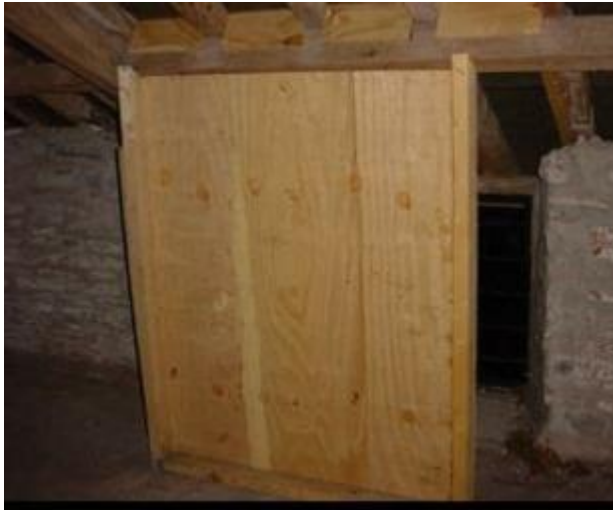
photo 8. showing a baffle to reduce drafts
