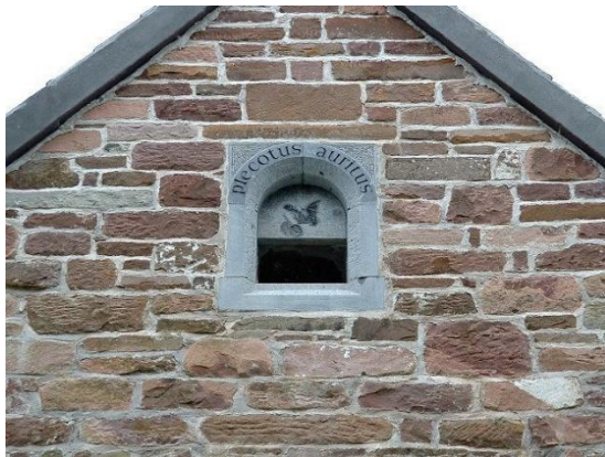
Photo 6. Example of a gable access point for Brown long eared bat which would suffice for Lesser horseshoe bat.
