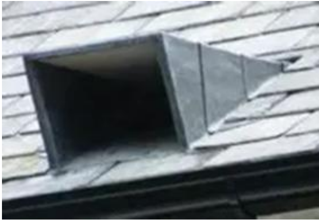
Photo 7. showing alternative access in roof for Lesser horseshoe bats to access loft space.
