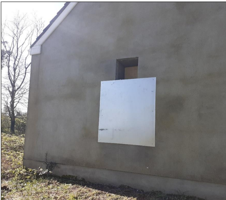
Plate 1c: Ballykilty Bat House, Co. Clare – please note the lead sheet below the entrance point to reduce Pine Marten entering the structure.
