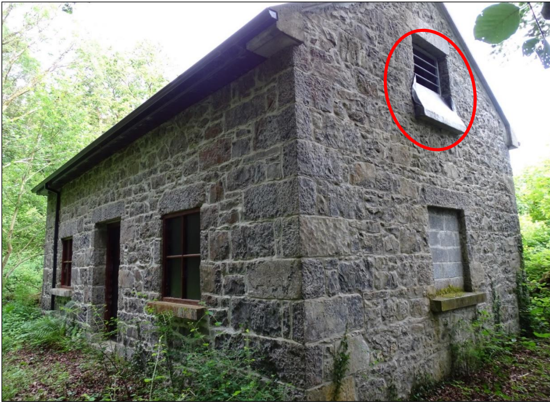
Plate 1b: Garryland Lodge LHB Roost, Garryland Nature Reserve, Gort, Co. Galway – please note the lead sheet around the windowsill to reduce Pine Marten entering the structure.
