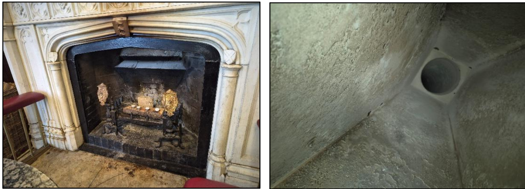
Plate 34: Chimney in the cocktail bar inspected for signs of bat activity.
