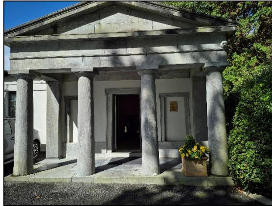
Plate 26: Gate Lodge exterior.
