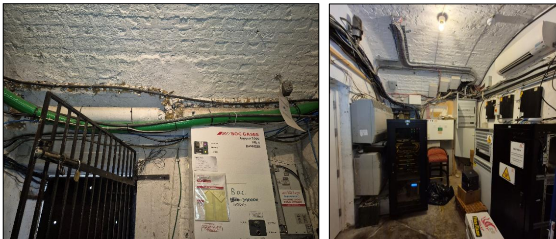
Plate 19: Basement area outside the wine cellar.
