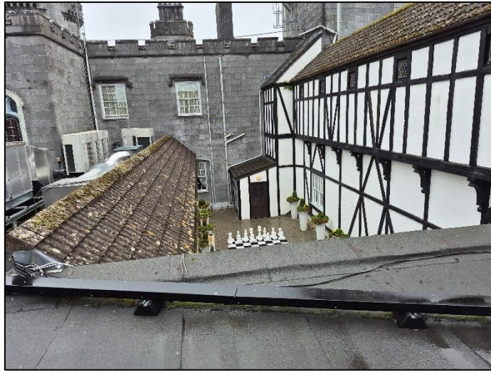
Plate 17: False roof overlooking the courtyard.
