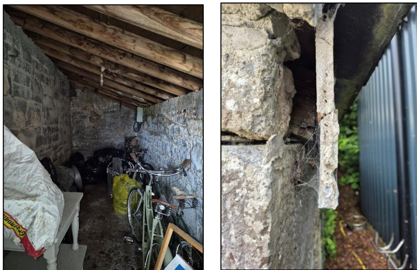
Plate 23: Lean-to shed interior (Left) with visible access point (Right).
