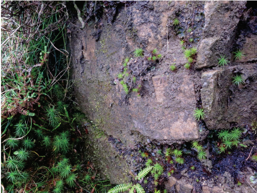
Photograph 3: Damp face of siliceous rock, on which B. trichodes grows.
