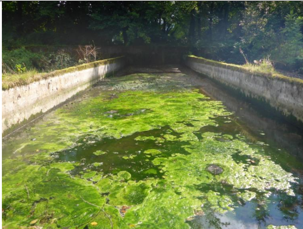
Photo 8.25 Bay 2 header tank at Site 2 is slower to empty.
