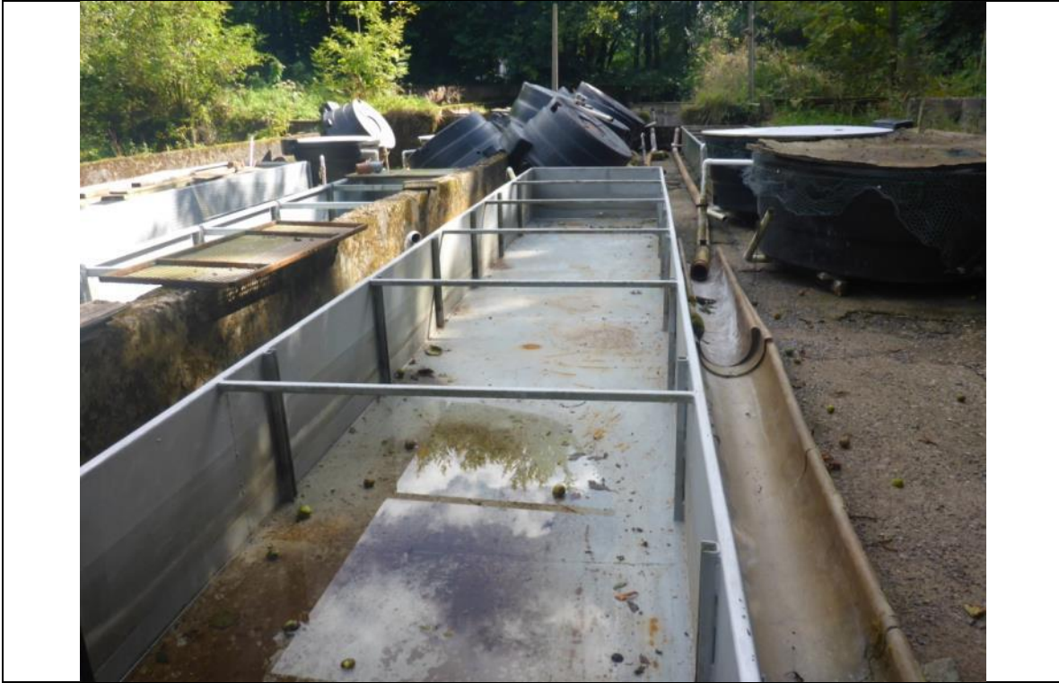
Photo 8.23 the cleaned site at Site 2.
