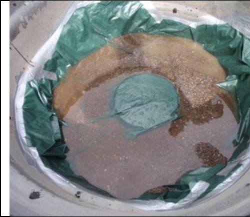
Photo 6.5 Lined and gravelled tank being watered, 2014
