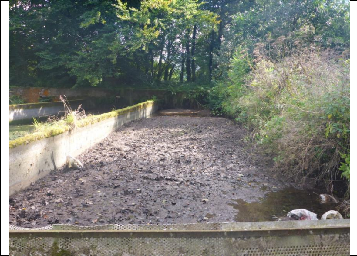
Photo 8.24 Bay 1 header tank at Site 2.
