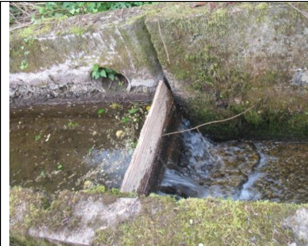
Photo 6.1 Channel with removable weir structures at Site 2
