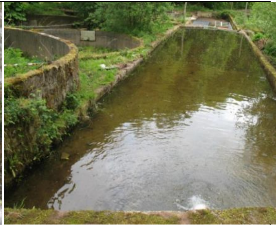
Photo 6.2 Settlement pond above tanks in each bay at Site 2
