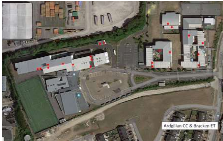
Plate 3.3 Ardgillan Community College/ Bracken Educate Together site adjacent to the Wavin plant
