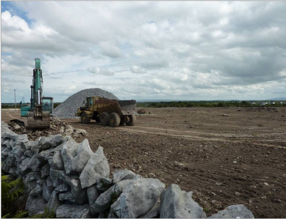
Plate 27 A large area (approximately 22ha) of land reclamation at Mountscribe, Co. Galway (NSLP32).
