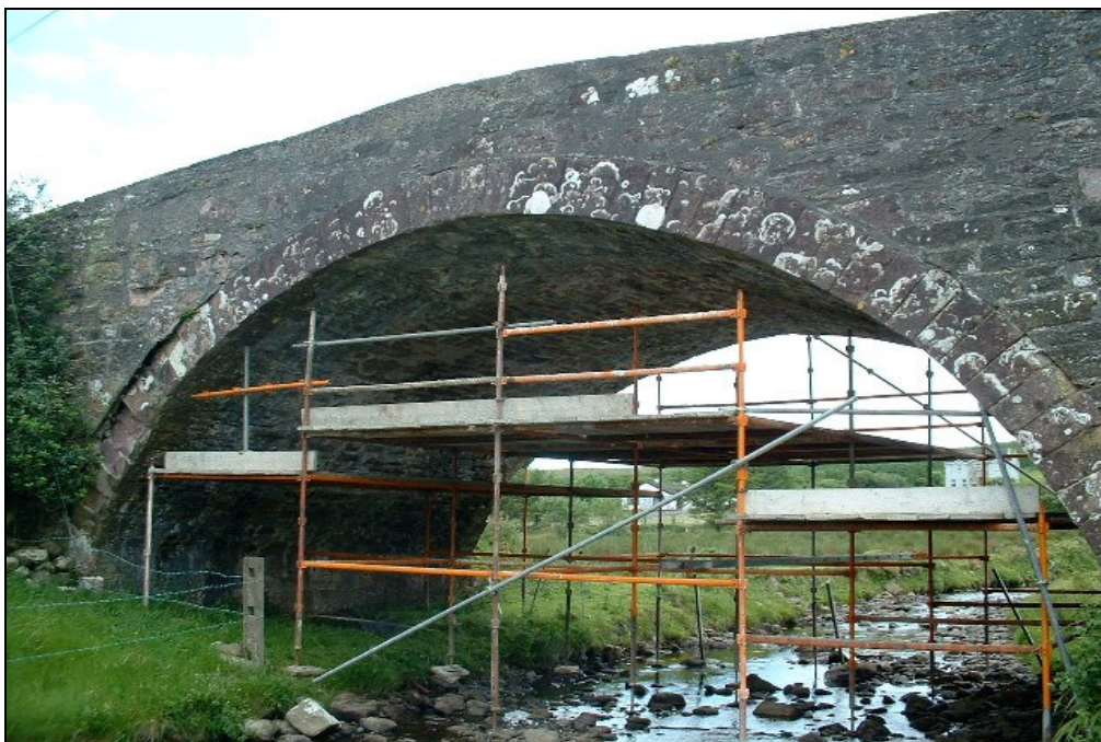
Figure 17. Bridge repair works which may impact bat roosting sites
