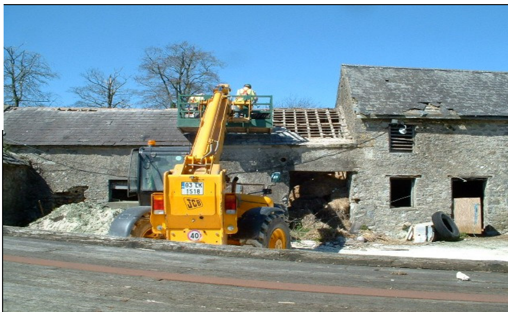
Figure 19. Removal of older buildings with potential as bat roosting sites
