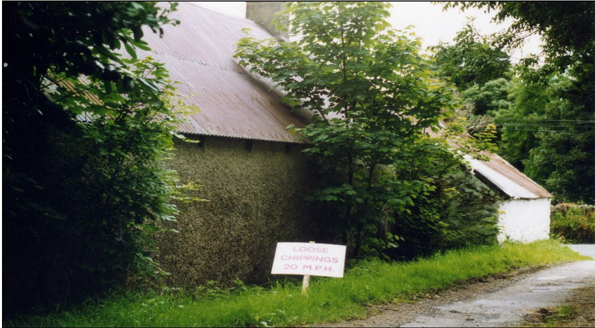
Figure 9.2.1 Affick cottage and shed before renovation
