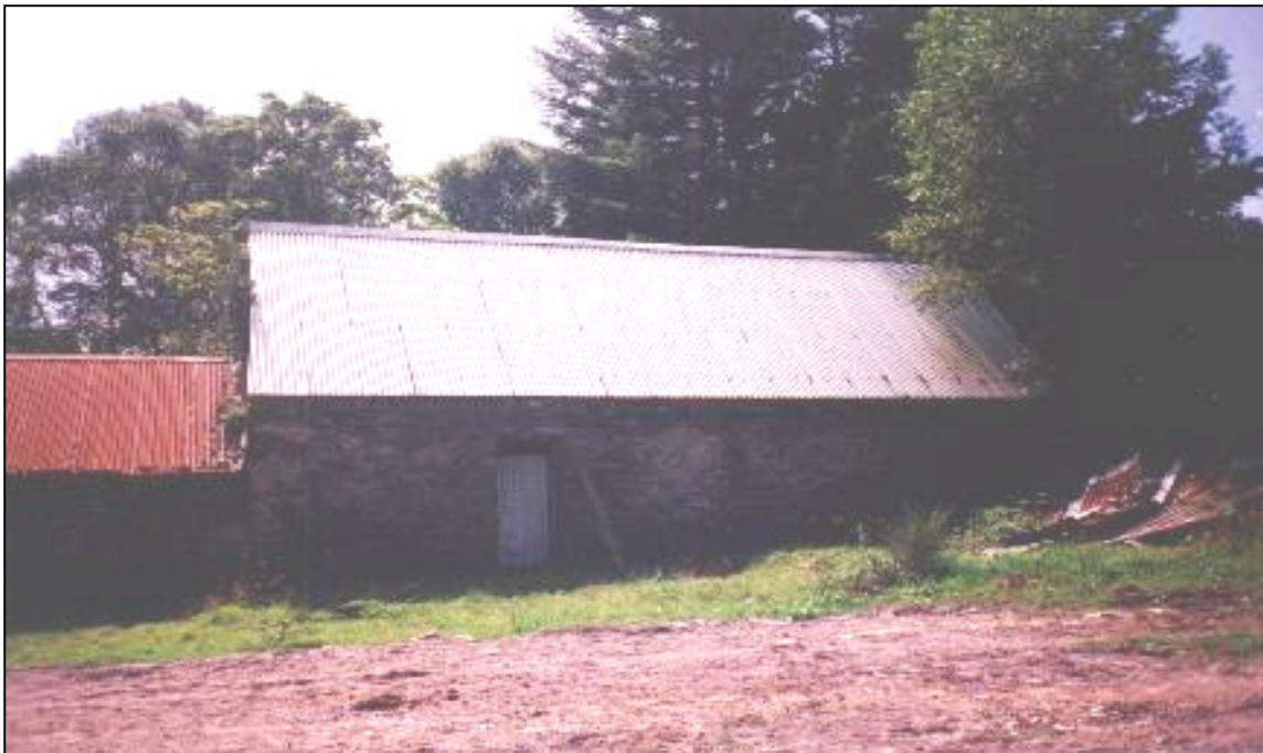
Figure 9.3.1 Blackwater Bridge lesser horseshoe roost after new roof was fitted.
