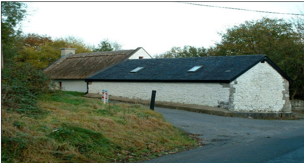
Figure 9.2.2 Affick cottage after renovation
