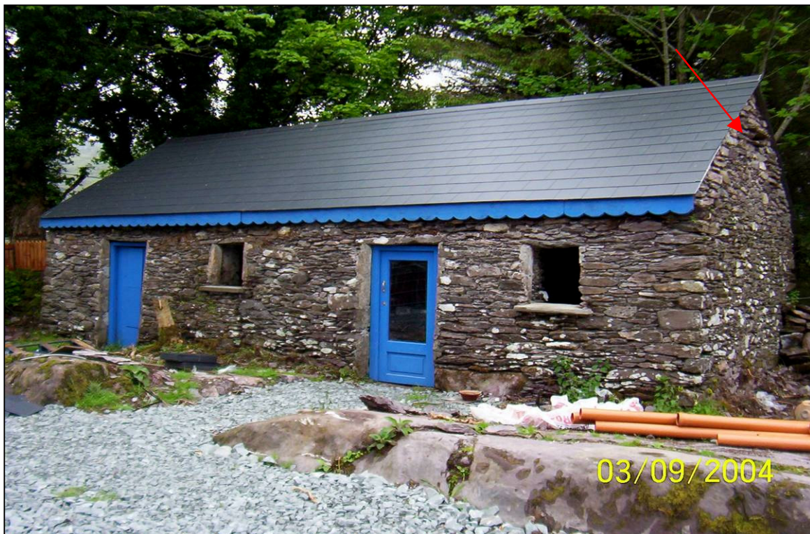
Figure 9.7.1 Glaninchiquin outbuilding during renovation. Bat access highlighted.
