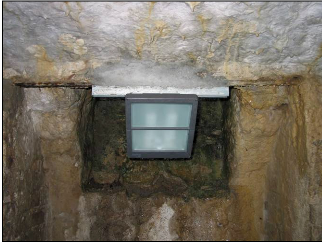
Figures 9.8.1 & 9.8.2 Lighting installed within tunnels.
