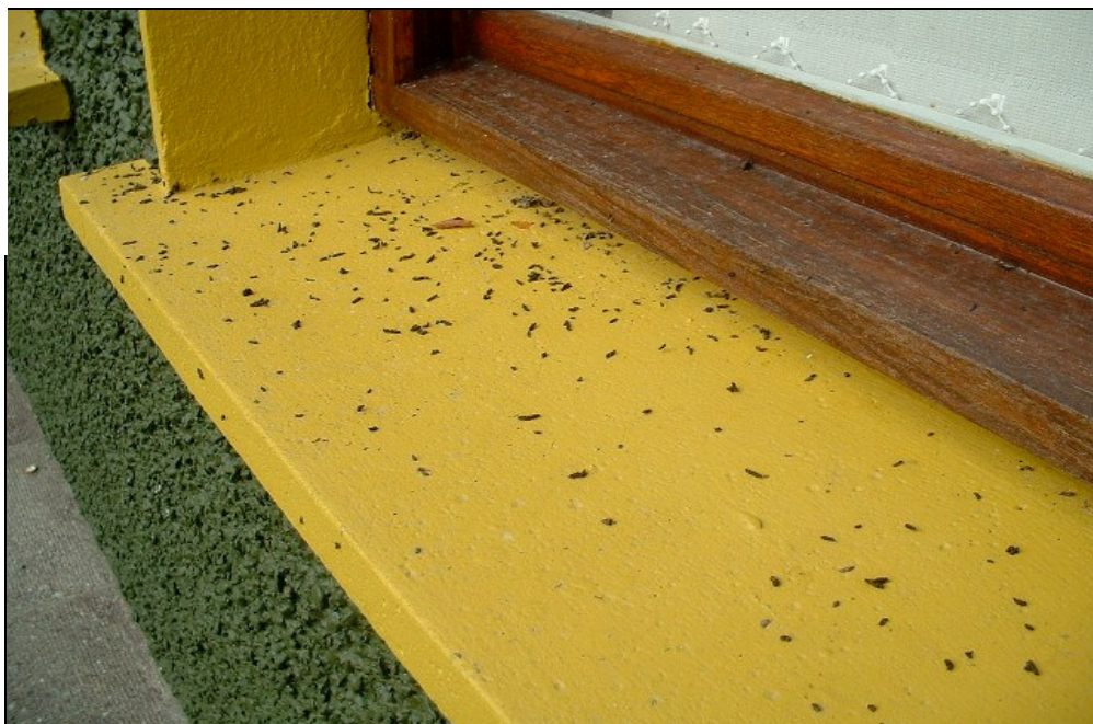
Figure 16. Pipistrelle droppings on window sill beneath roost access point
