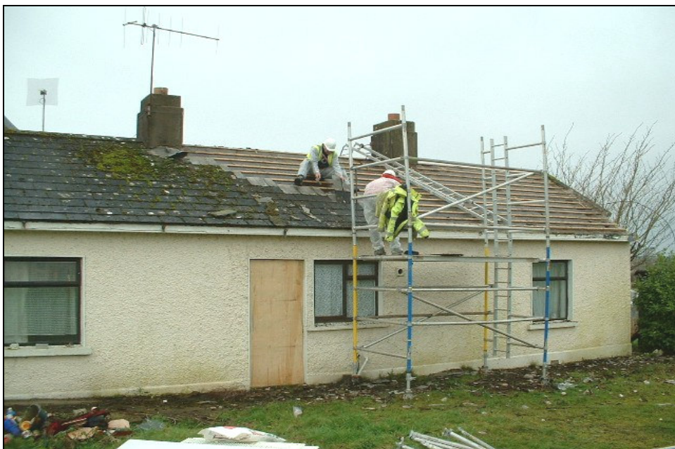
Figure 25. Re-roofing operations may require timing restrictions
