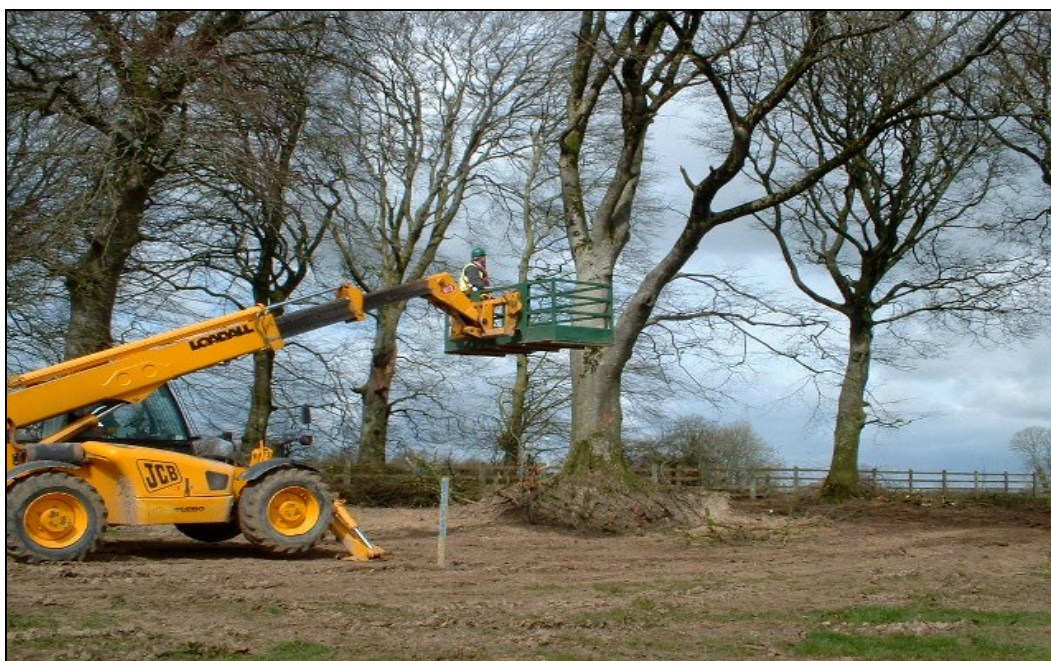
Figure 1. Tree removal by manual dismantling to safeguard bats
