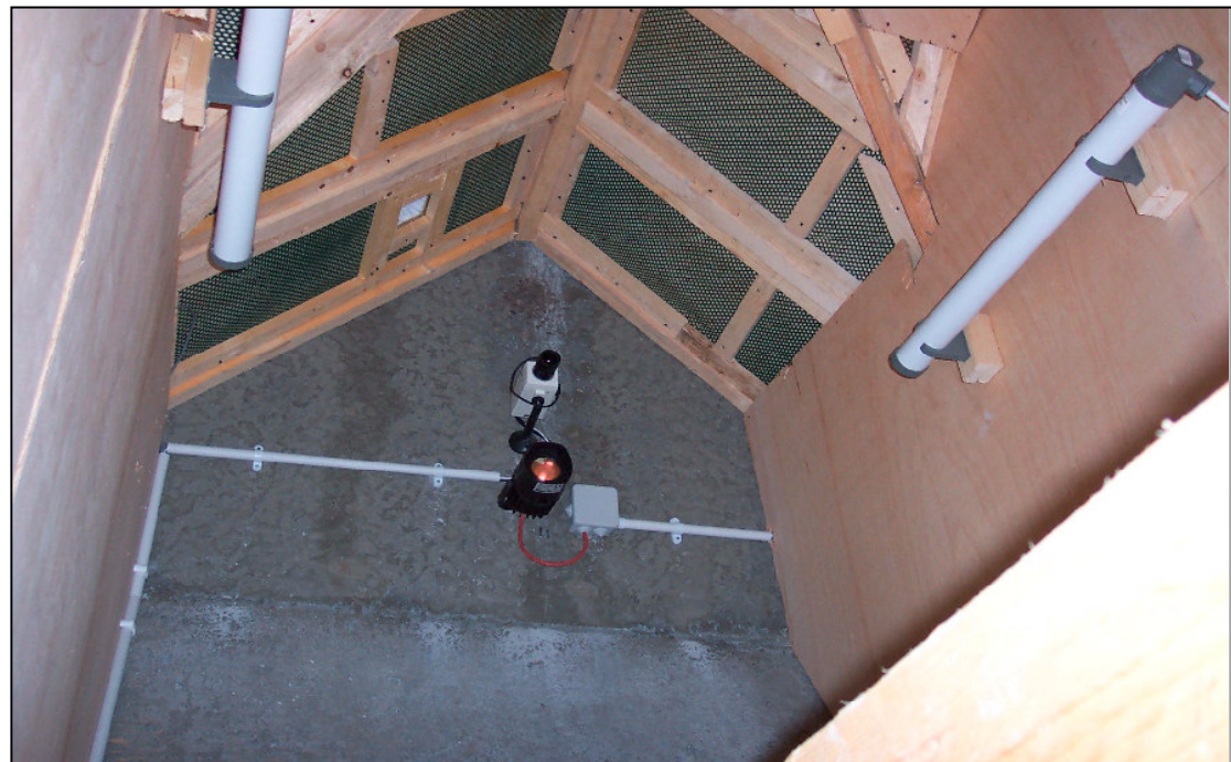
Figure 29. Roof apex of bat house showing two thermo- statically controlled infra-red heaters and remote controlled CCTV monitoring system
